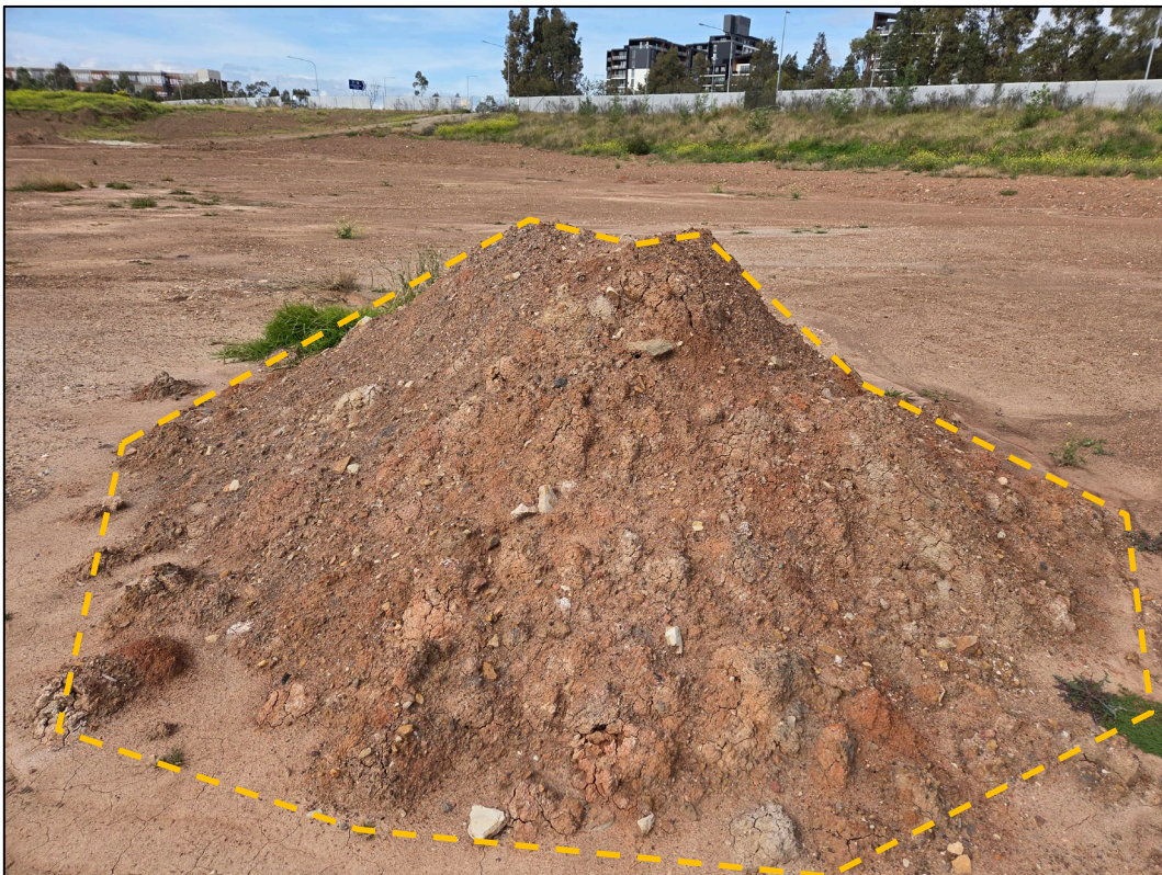
Site Photograph 6.8.2 View of the stockpiled fill material located central of the northern portion of Lot 9 in DP1275478, as observed facing north on 8 August 2025.
