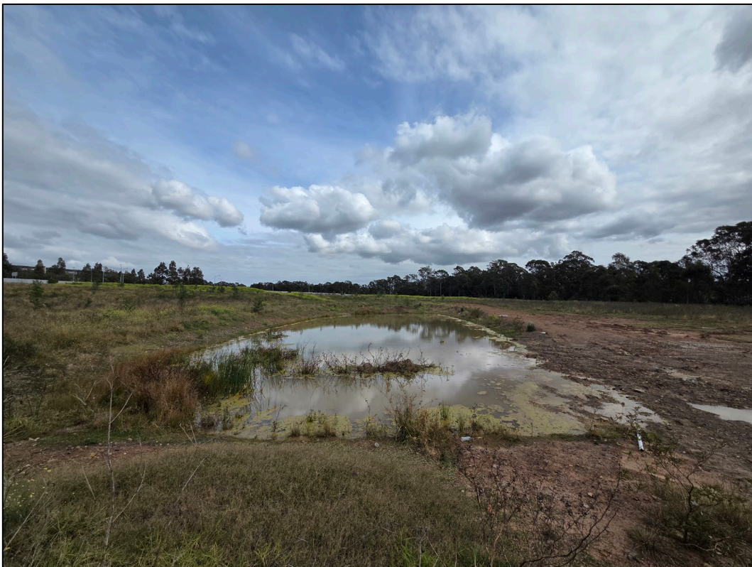
Site Photograph 6.2.5 Representative view of the sediment basin encountered within Lot 103 DP1275550, as observed facing west on 8 August 2025.
