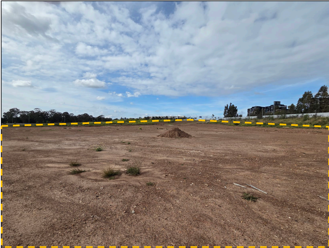
Site Photograph 6.8.1 View of the fill materials observed within northern portion of Lot 9 in DP127547, as observed facing south on 8 August 2025.
