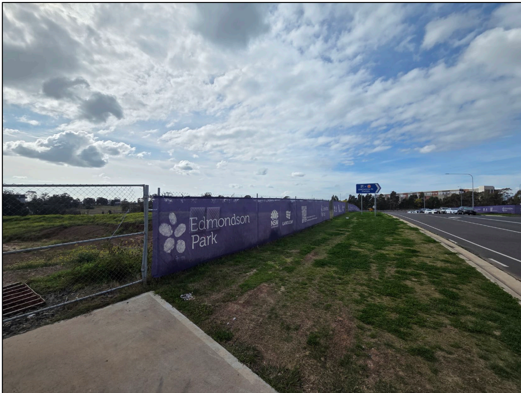
Site Photograph 6.3.1 Representative view of the boundary fencing along northern portion of Lot 9 in DP1275478 and Lot 103 & 104 in DP1275550, as observed facing east on 8 August 2025.
