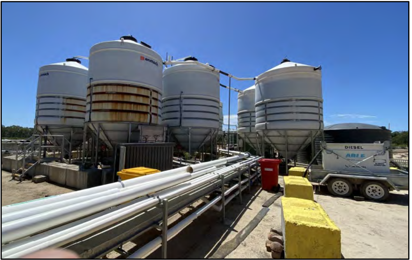
Photoplate 5. Water Recycling Plant
