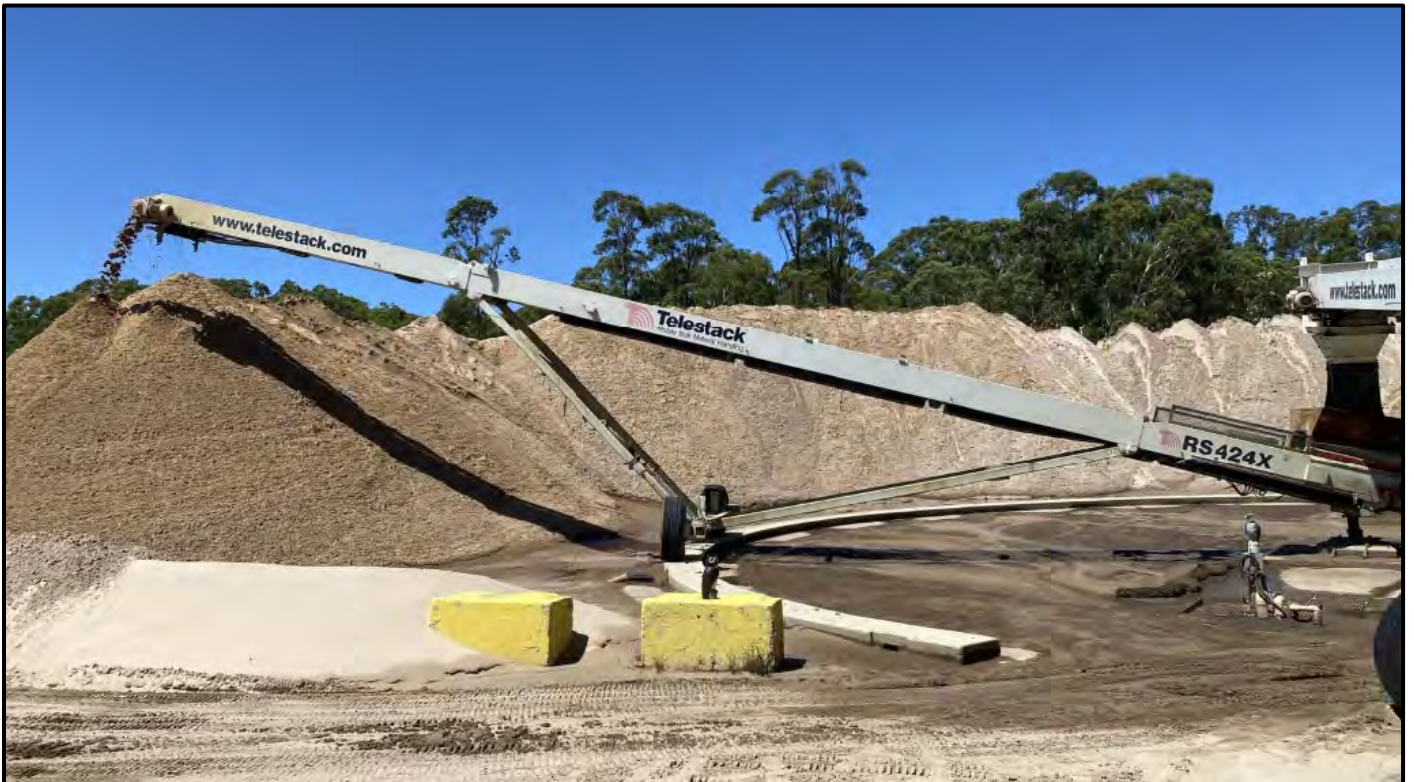
Photoplate 4. Washed Sand Stockpiling
