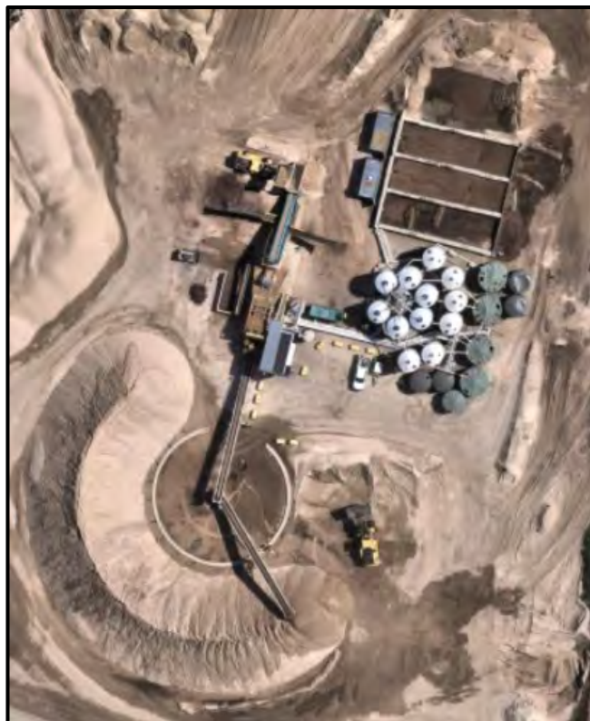
Photoplate 2. Existing Cabbage Tree Sand Quarry Processing Plant Overview
