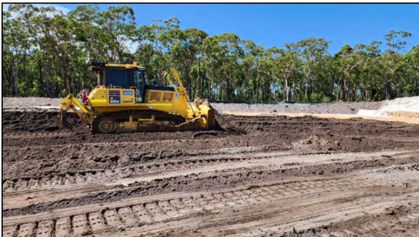
Photoplate 6. Spreading of Topsoil on Pit Floor at Cabbage Tree Sand Quarry
