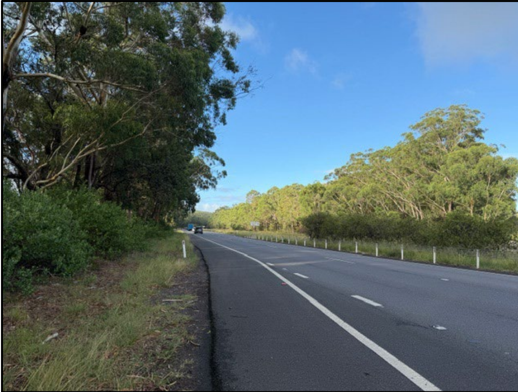
Photo 1 – View along Nelson Bay Road south-west of the site in the vicinity of the proposed deceleration lane
