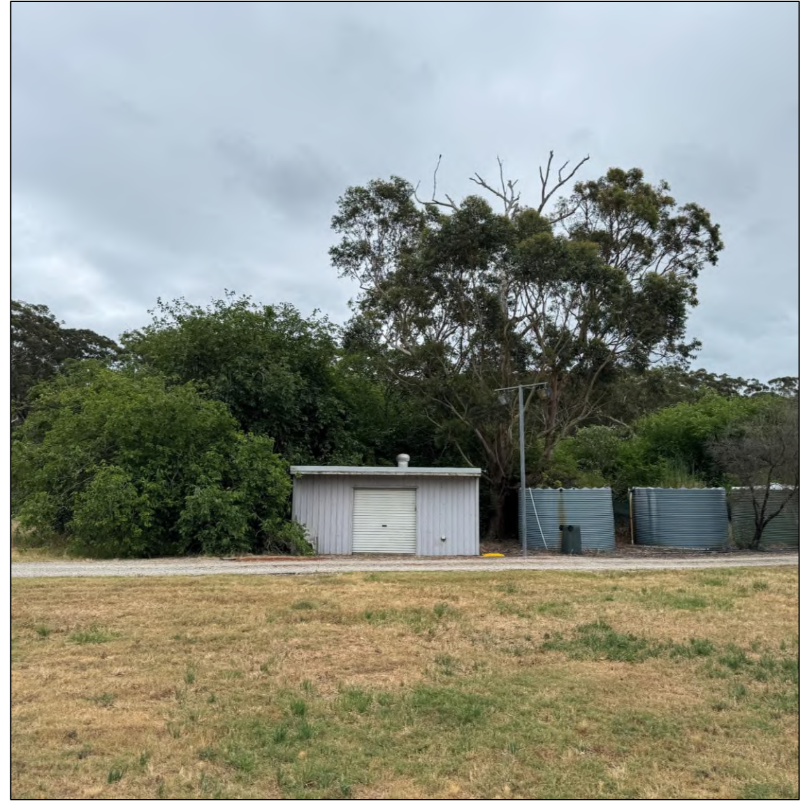
Photo 4 – Shed, water tanks, driveway, overground vegetation.
