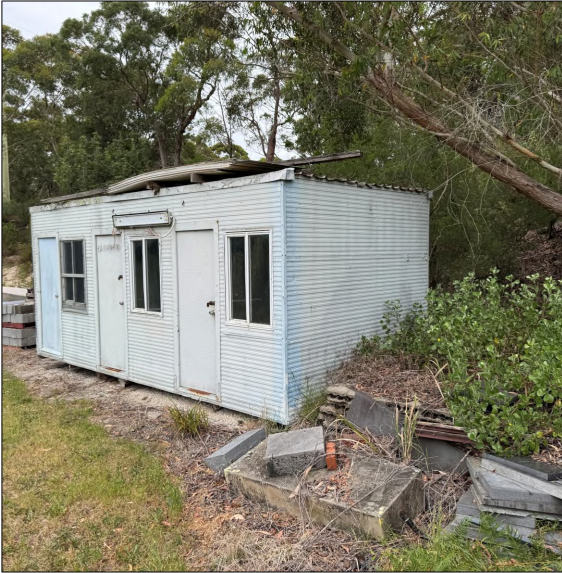
Photo 7 – Shed, building material stockpiles.
