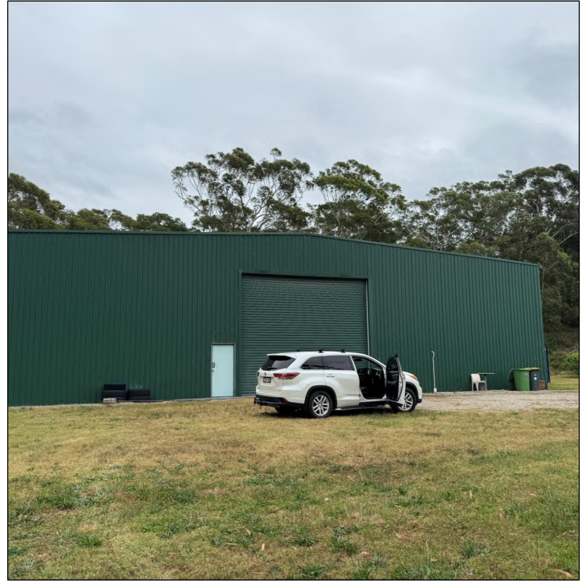
Photo 6 – Large shed (workshop, machinery storage)
