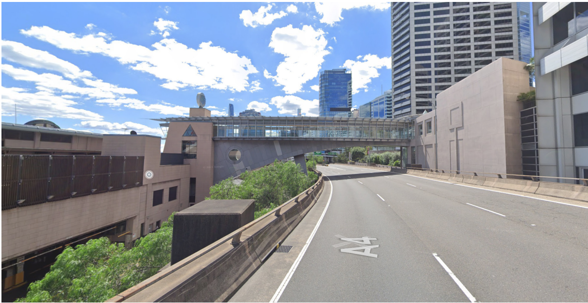
3. Current bridge connection between the Darling Park development and the existing Cockle Bay Wharf.
