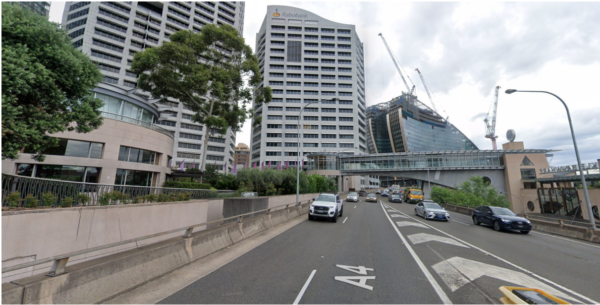
1. Existing conditions with the Western Distributor running right neext to the existing sites.
