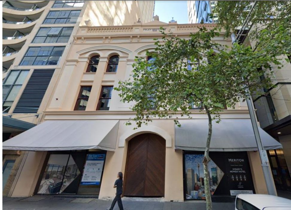
Figure 30: Former “Foley Bros” warehouse at Sussex Street.
