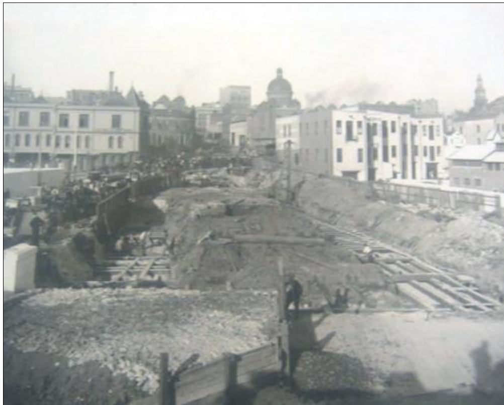
Figure 7: Photograph of the Sydney Approaches from the Album of Percy Allen, dated 2 May, 1900. Department of Commerce, cited in Otto Cserhalmi + Partners, Pymont Bridge Darling Harbour, Sydney, Conservation Management Plan, 2006.
