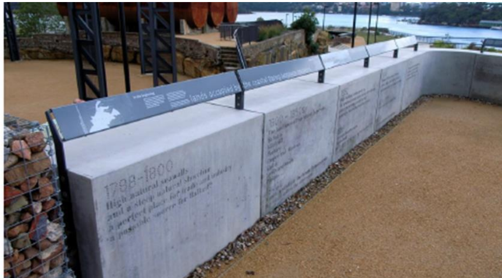
Figure 35: The display panels used in this heritage interpretation for Ballast Point consists of concrete section with timeline history information. The display serves as a retaining wall as well as a display. This could potentially be used along the foreshore, in some areas
