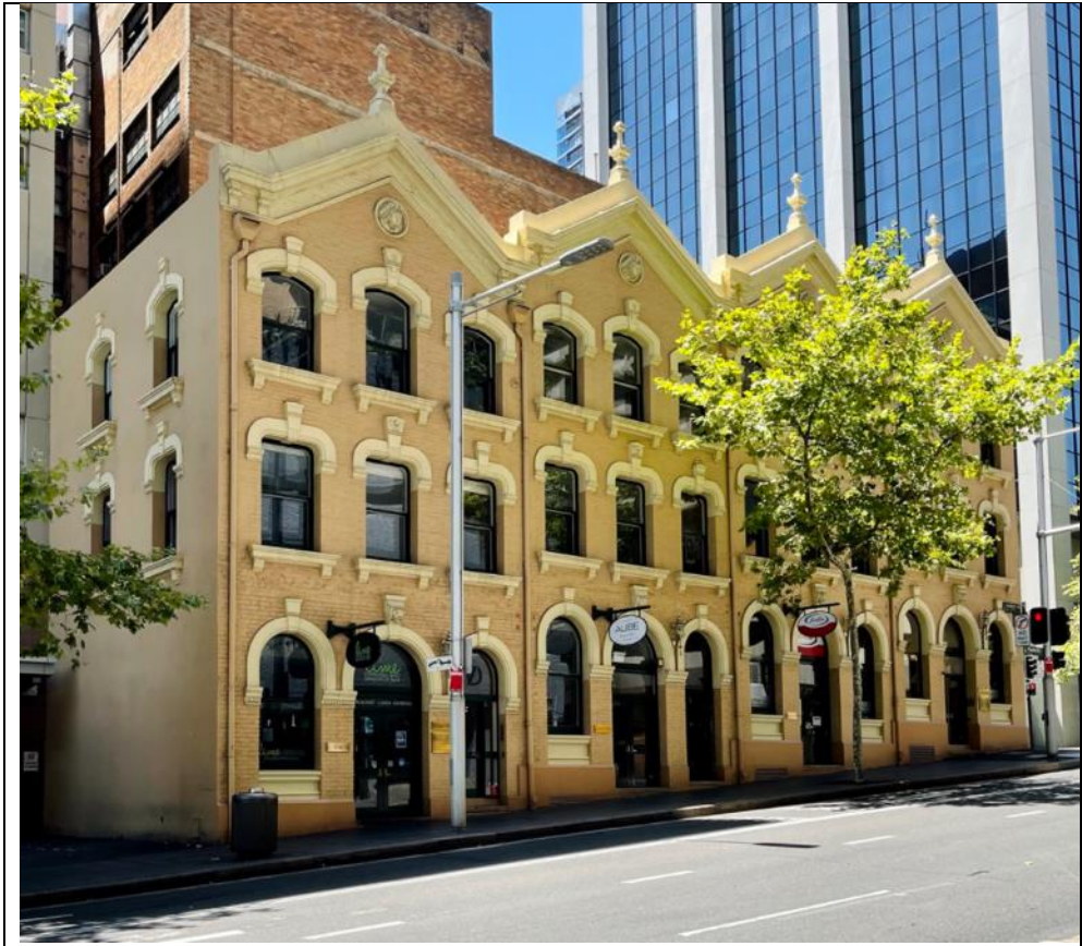
Figure 32: Archway terrace viewed from Market Street.
