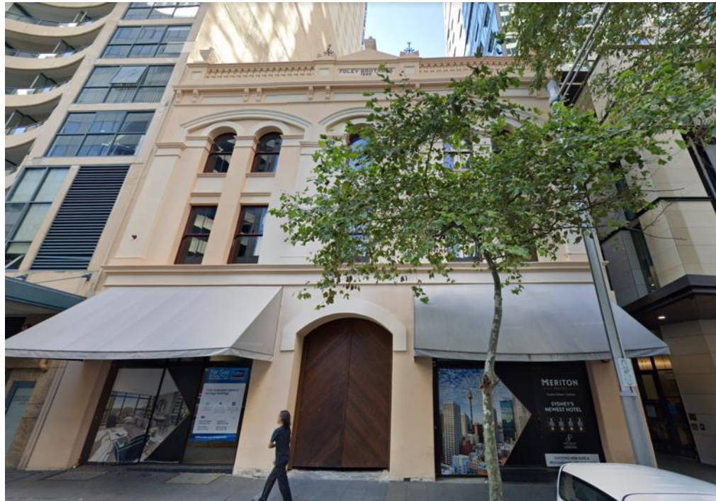
Figure 25: Former “Foley Bros” warehouse at Sussex Street.
