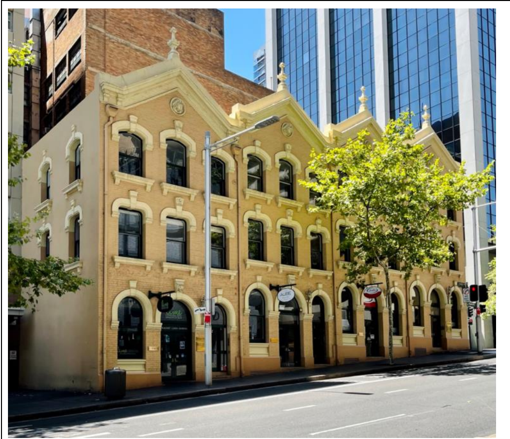
Figure 27: Archway terrace viewed from Market Street.
