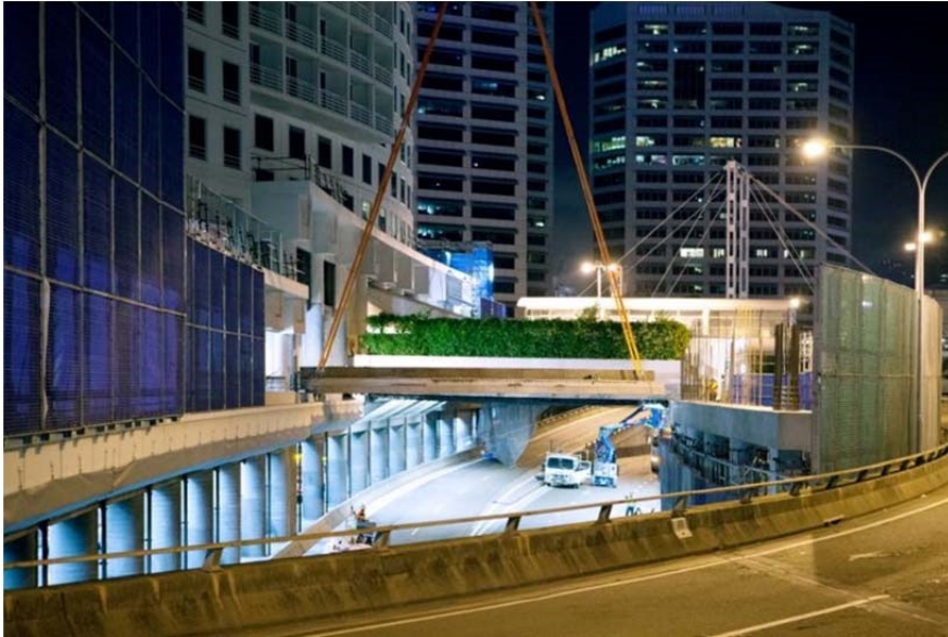
Figure 19 Night works at the 161 Sussex Street development. Multiplex has experience craning precast beams into position over the Western Distributor.
