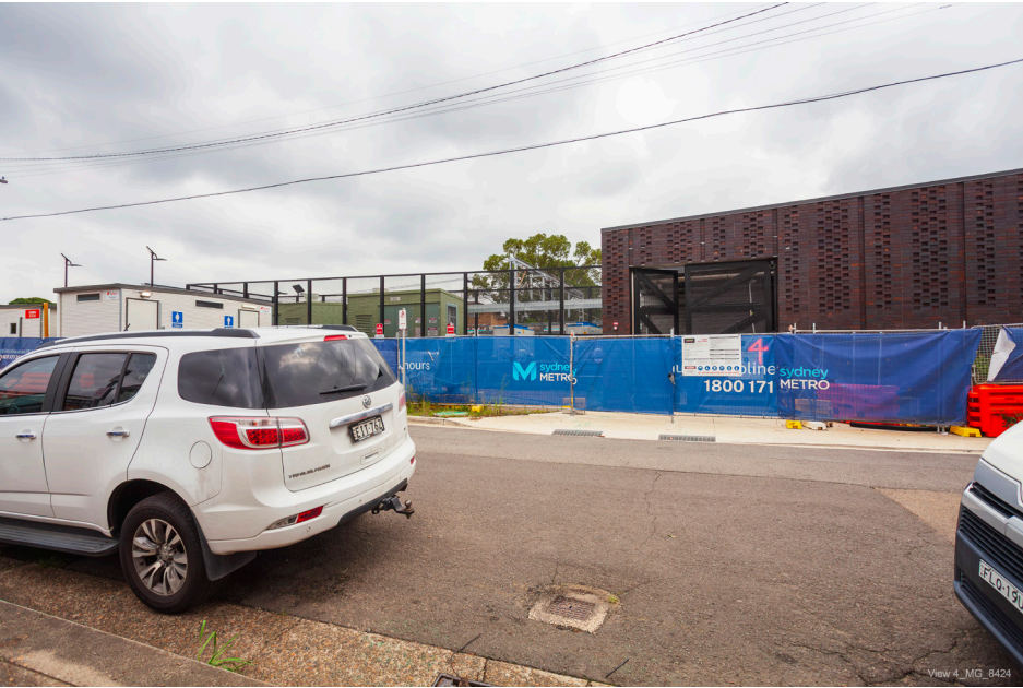
View 4_MG_8424 - Existing
