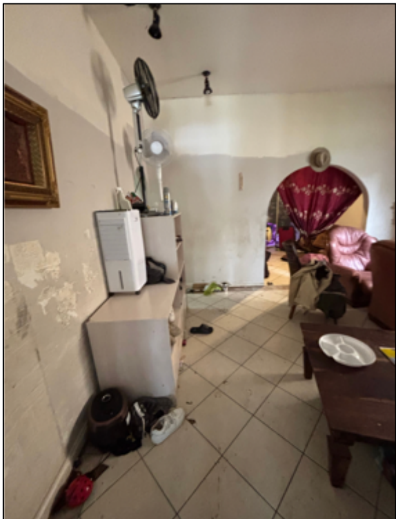
Figure 21. Internal view of 30 Campsie Street.
