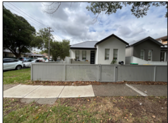
Figure 17. View from Campsie Street facing south showing 26 Campsie Street.
