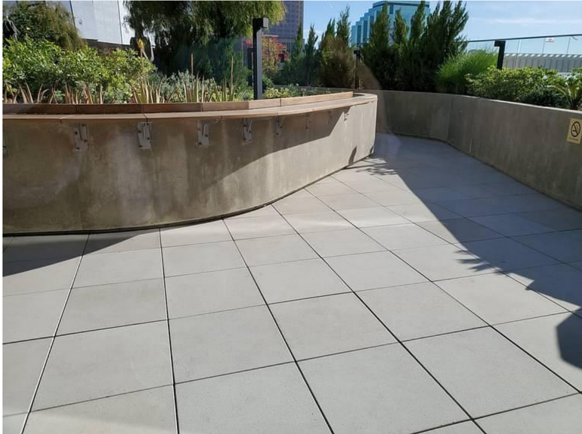
Figure 4 Roof Terrace Pavements with High SRI Materials
