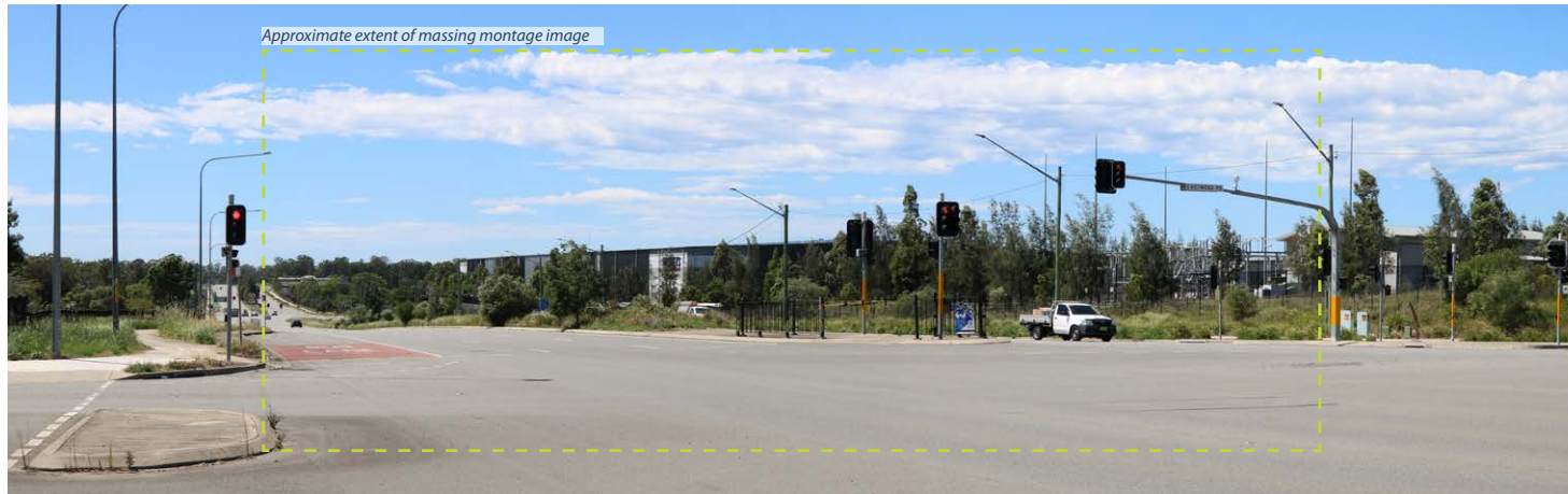
Image 15 Photo stitched view south-east towards site (NOTE: Photo stitching provides a level of distortion to photographs, but is used in this instance to establish context).
