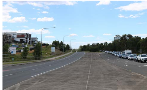
Image 10 Camden Valley Highway
