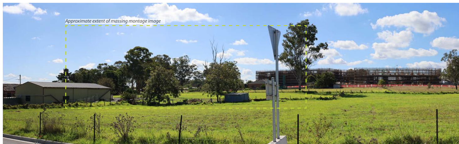
Image 23 Photo stitched view north towards site (NOTE: Photo stitching provides a level of distortion to photographs, but is used in this instance to establish context).
