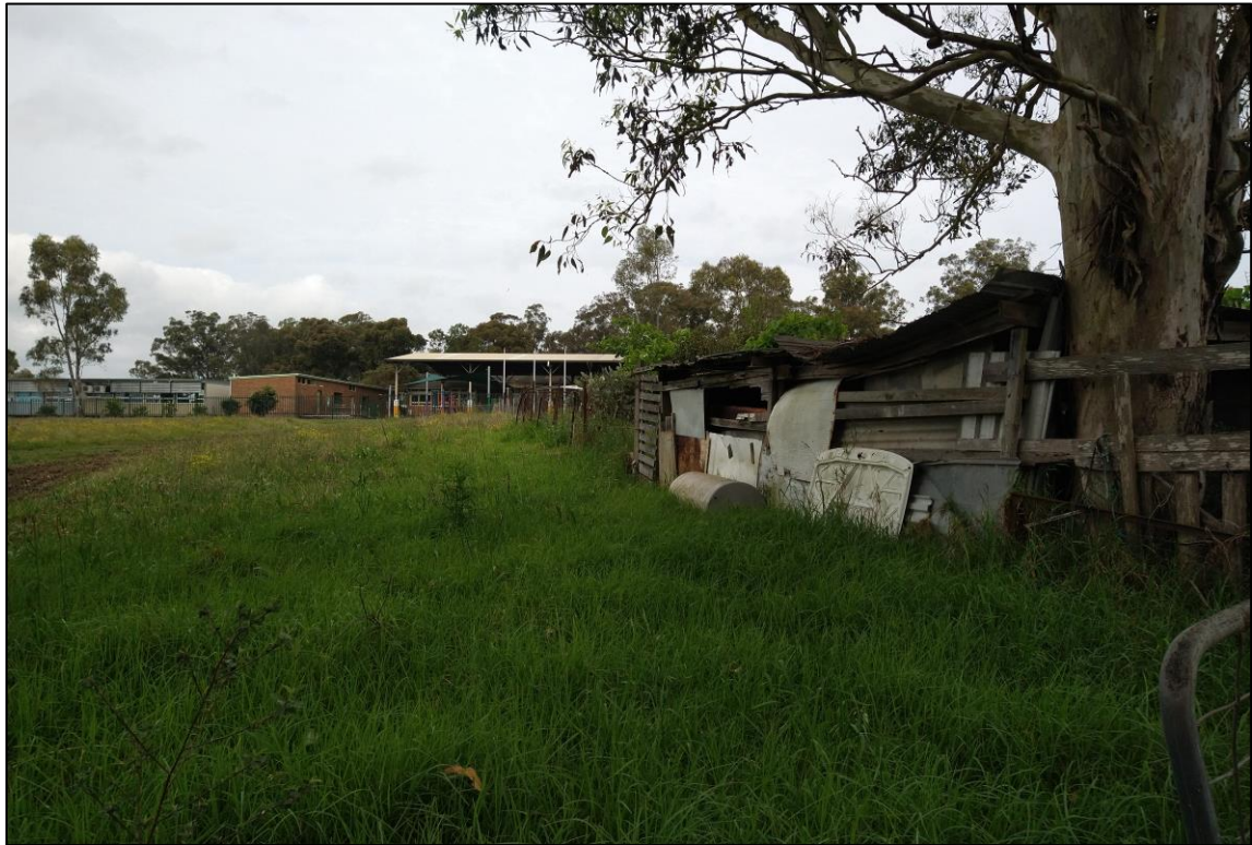
Photograph of Sheds in south of site property of Site of potential contamination.
