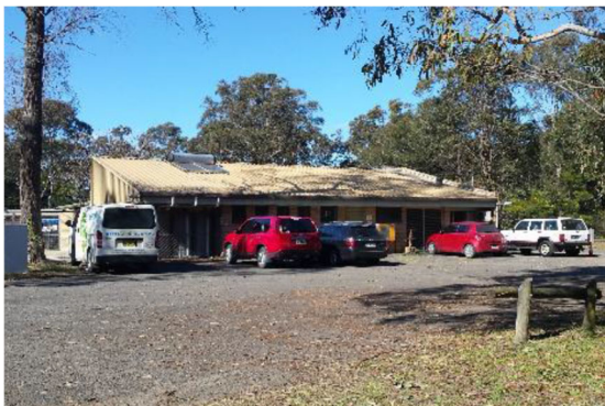
Photo 4.1 Main animal shelter building and car park
