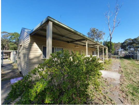
Photo 4.3 Colorbond cladded building
