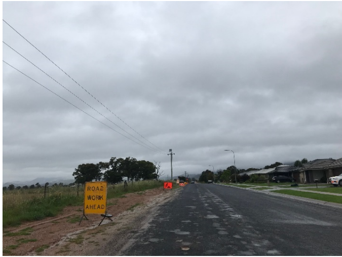
Photo 5 – Traffic controls – ‘Road Work ahead’ sign
