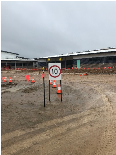
Photo 7 – Speed limit of 10km/h at the entrance of the site
