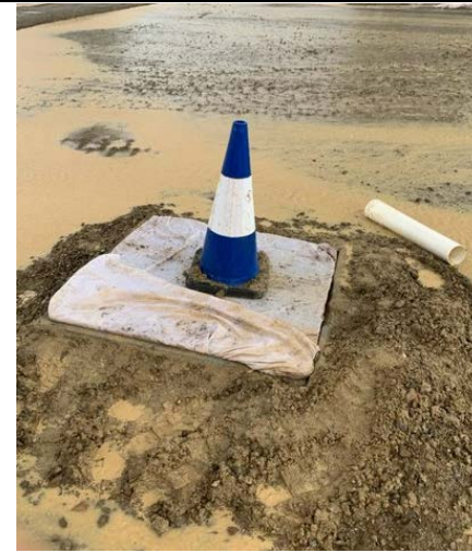
Photo 10 – Carpark pits protected
