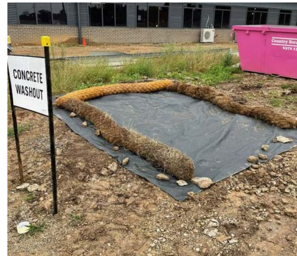
Photo 12 – Concrete Washout area maintained
