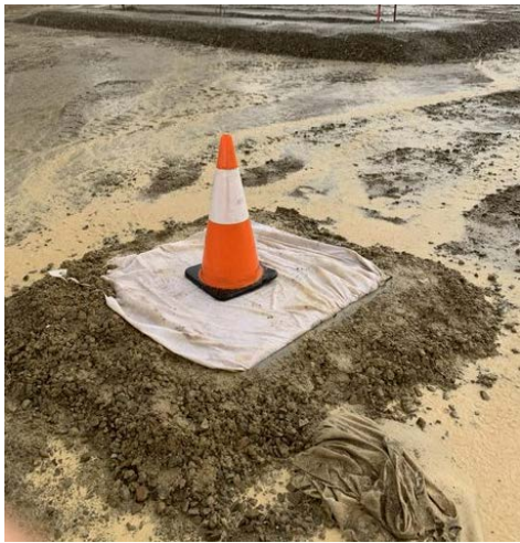
Photo 9 – Carpark pits protected
