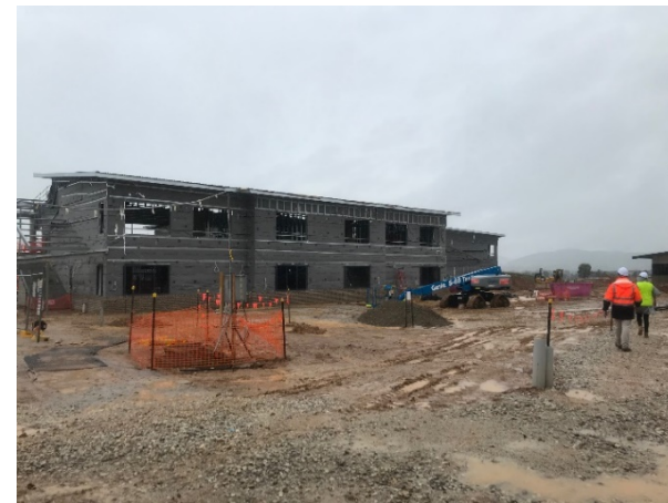
Photo 16 – Building structure and roof and walls sheeting completed
