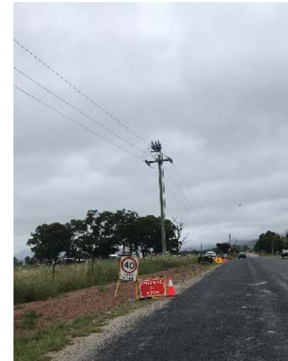
Photo 6 – Traffic controls - Speed limit sign 40km/h on Broadhead Rd
