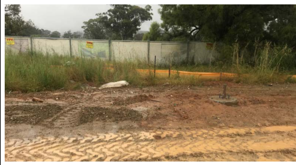
Photo 8 – Silt fence in place around the perimeter of the site
