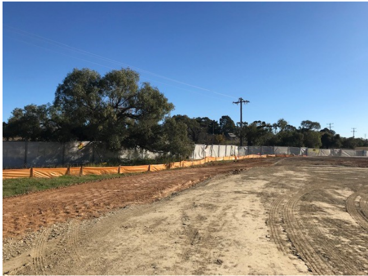
Photo 5 – Security fence and sediment fence installed around the perimeter.
