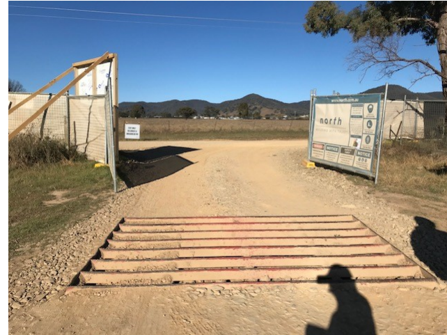
Photo 2 – Rumble grid in place at the site entrance/exit.
