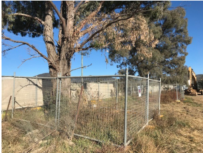
Photo 3 – Fencing around the trees installed.
