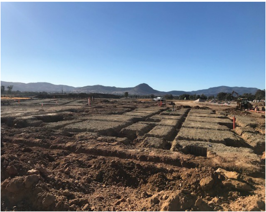
Photo 14– Drainage works and building foundations.
