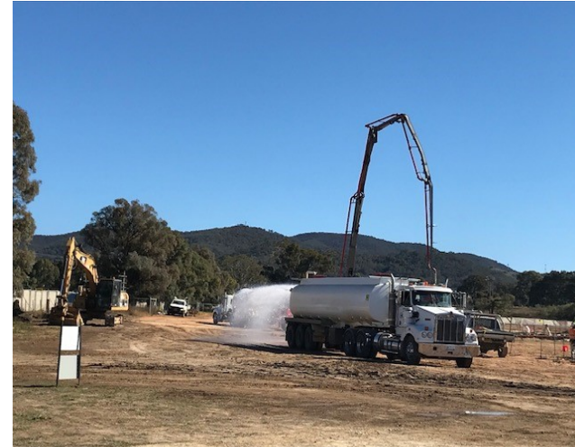
Photo 4 – Water cart was always available for dust suppression.
