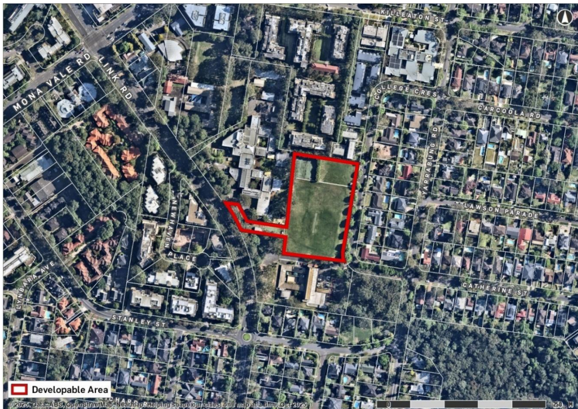
Figure 2 Aerial Photograph (Source: Urbis)
