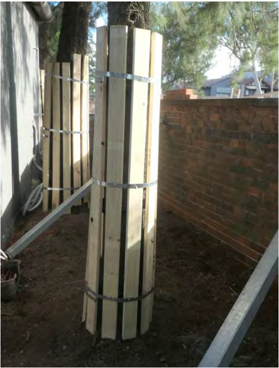
Example image of acceptable trunk protection battens
