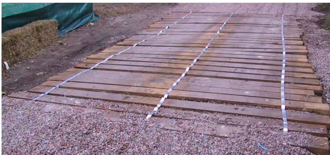
Figure 3.1 – Example of acceptable Tree Protection Area ground protection (Photo: Arterra)
