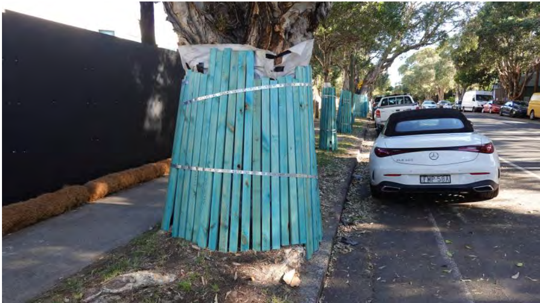
Figure 3.3 – Acceptable Trunk Protection batten installation – height of boards to be at least 2.4m or to the first branches. (Photo: Arterra)
