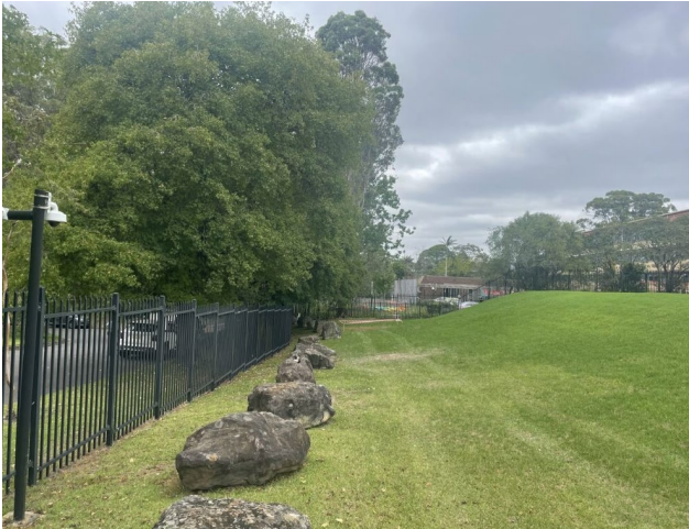
Figure 35 – View south along eastern boundary of the site, showing slope from level of playing field down to College Crescent
