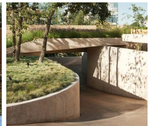
Level change - driveway and basement entry
