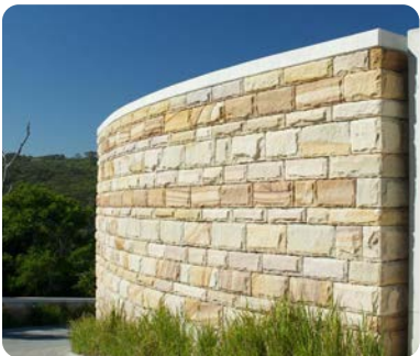
School Wall School perimeter HVM wall
