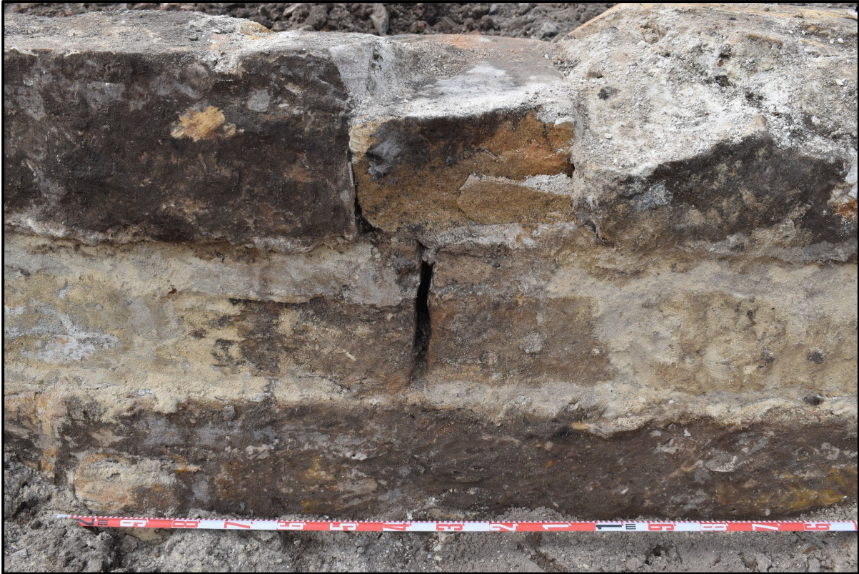
Figure 48. Weep hole in wall <007>
