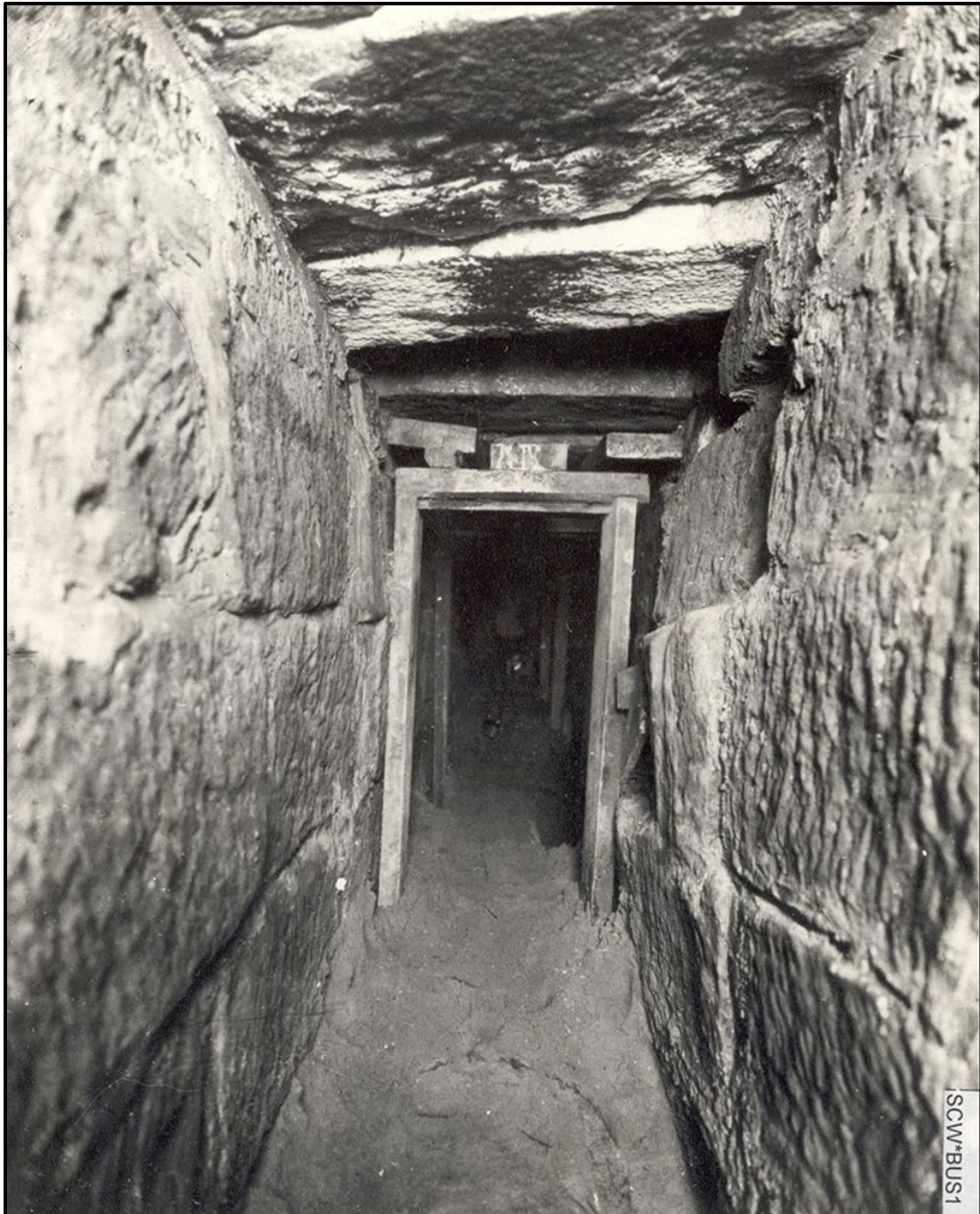
Figure 9. Busbys Bore at the intersection of College and Liverpool Streets, constructed with stone masonry lining. Source: Sydney Water Archives. (Based on historical information only a small portion of the tunnel was constructed in this way).
