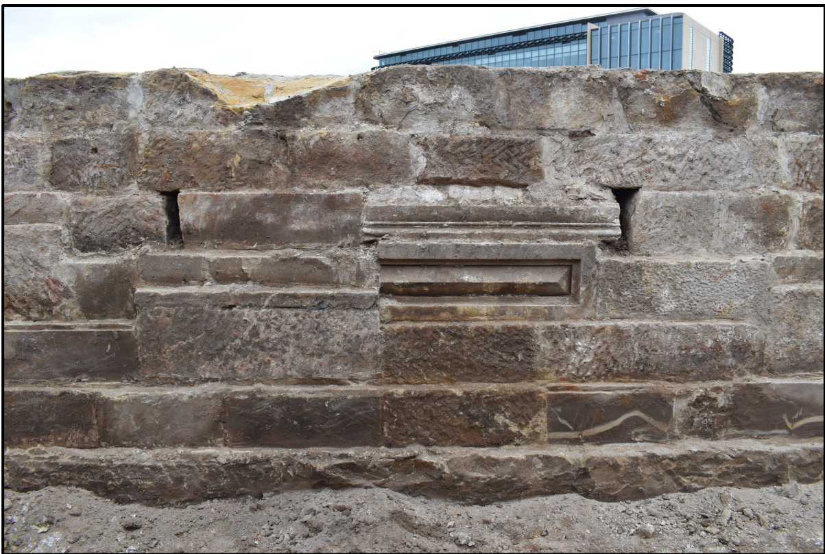
Figure 39. Weep holes and decorated stonework within <001>
