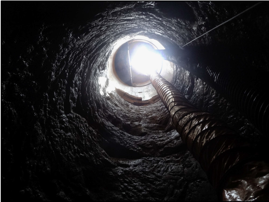
Figure 10. Busbys Bore Shaft 10 looking up showing dressed sandstone section of shaft (Source John Holland)
