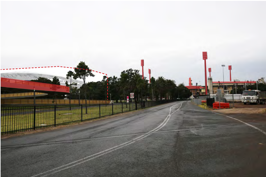
Original Photograph showing Alignment Points
