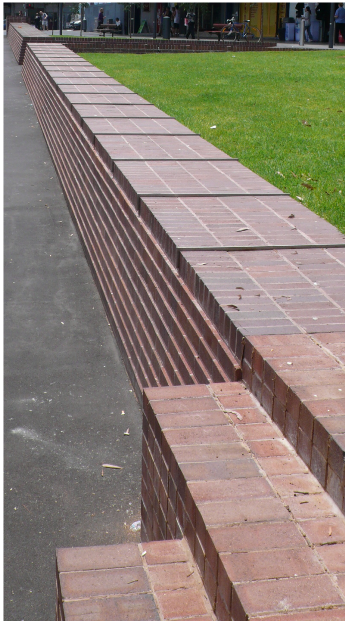
BWK(1) Medium Brown/Bronze Bricks (Exposure grade) - Exterior walls and podium plinth
