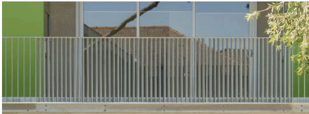
PC - White concrete architectural pre-cast concrete as diminishing balustrade upstand (BAL1) - Northern Balcony
