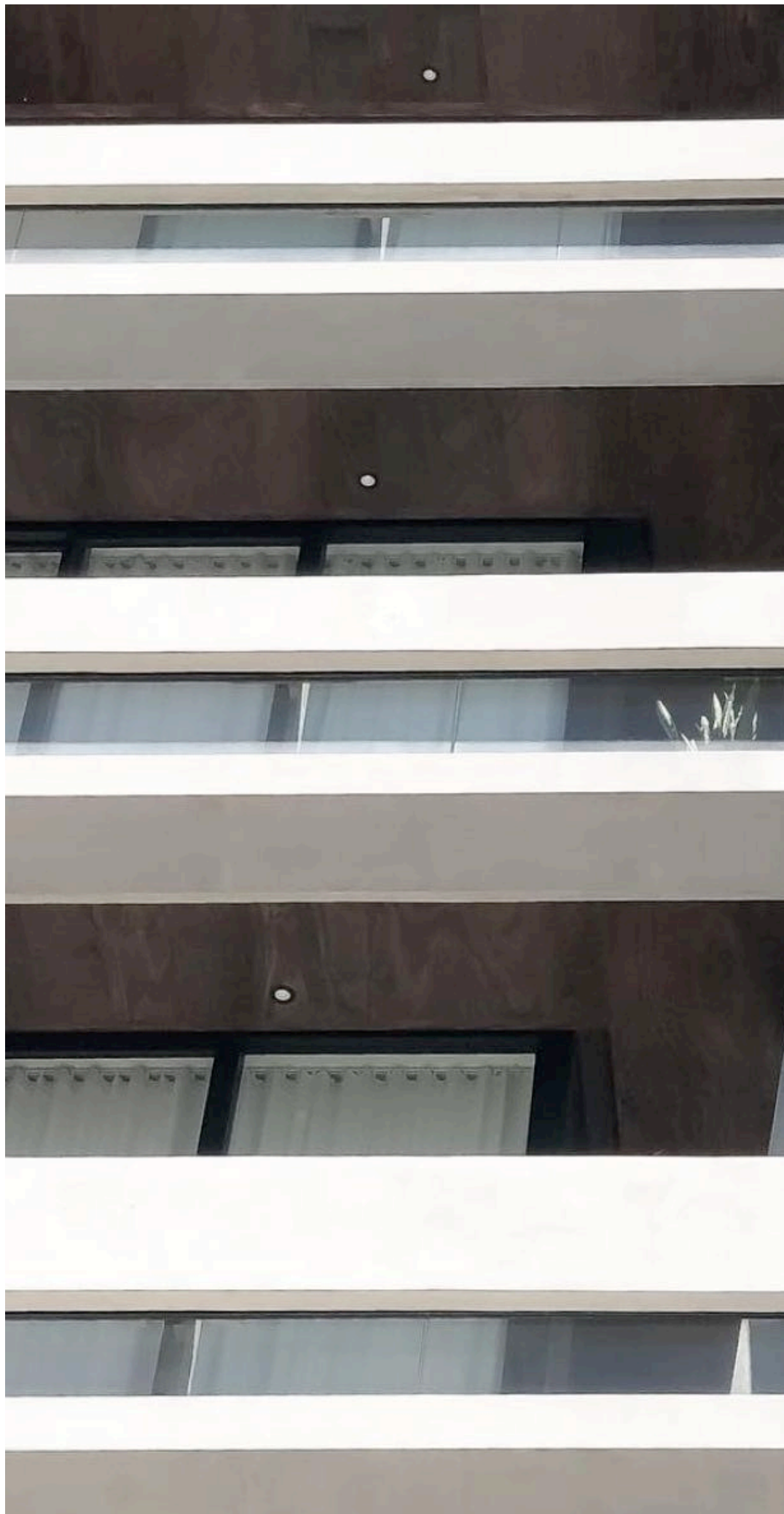
PC - White concrete architectural pre-cast concrete as diminishing balustrade upstand (BAL1) - Northern Balcony
