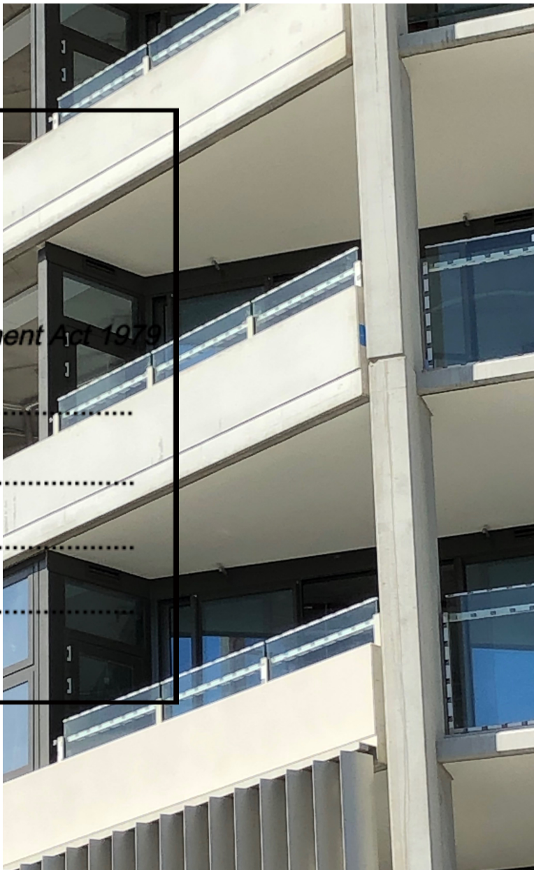
BAL(1) - Frameless glass balustrade fixed to back of white concrete precast upstand (PC) - Northern and South Balconies
