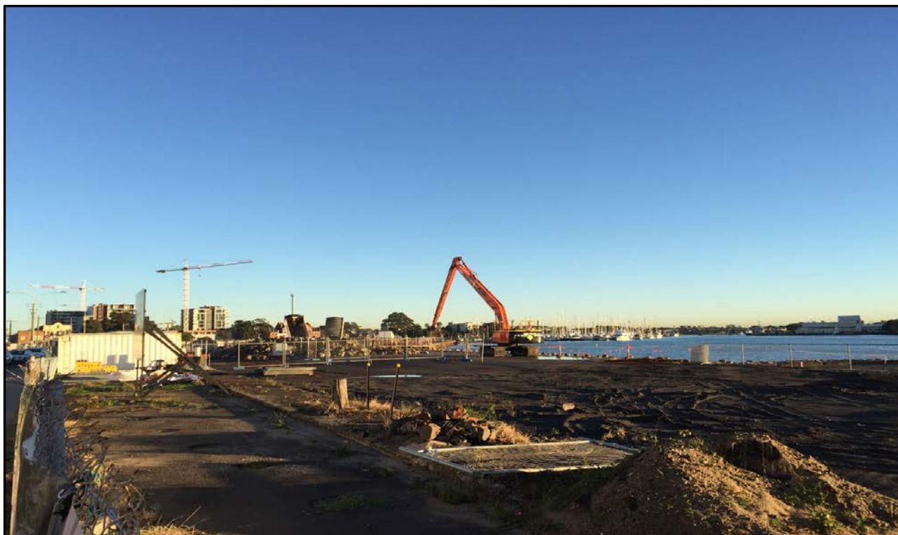
Figure 3 - Photo of the subject site looking north-west.
