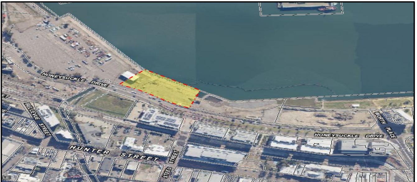
Figure 1: Lee 5 Development Site
