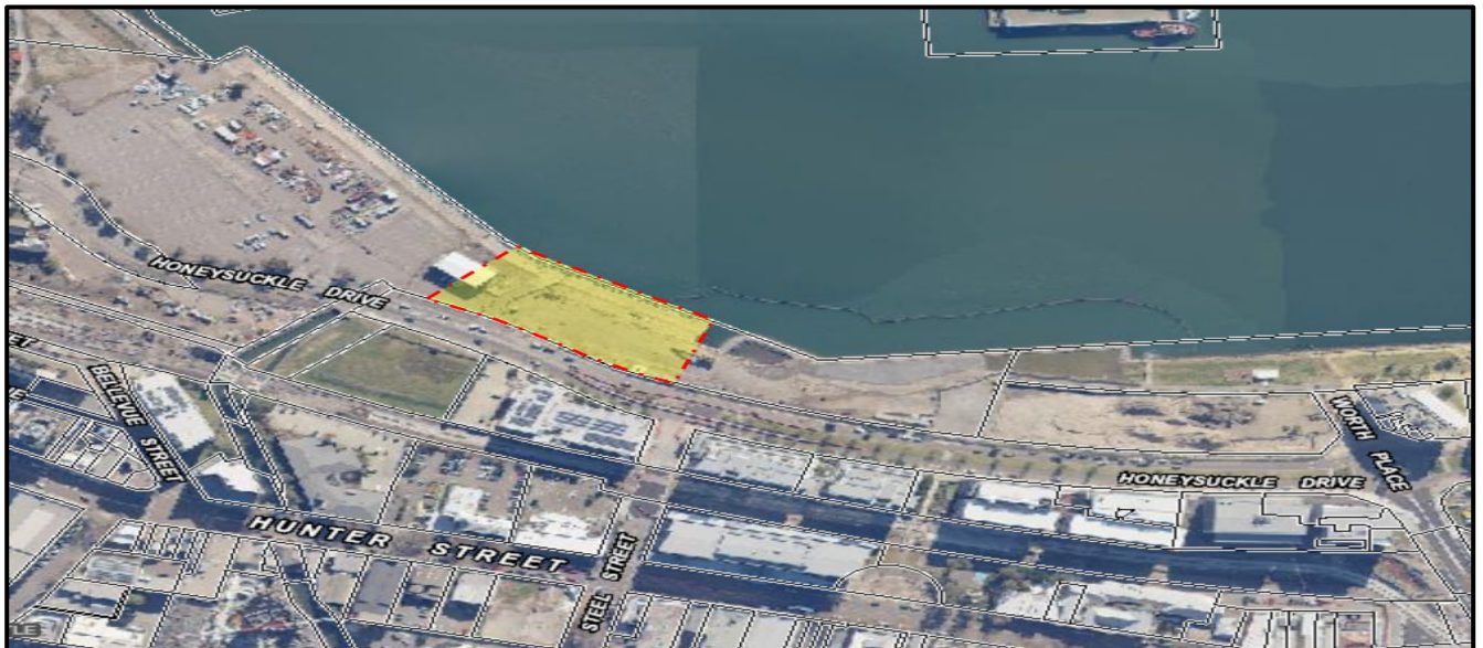
Figure 1: Lee 5 Development Site
