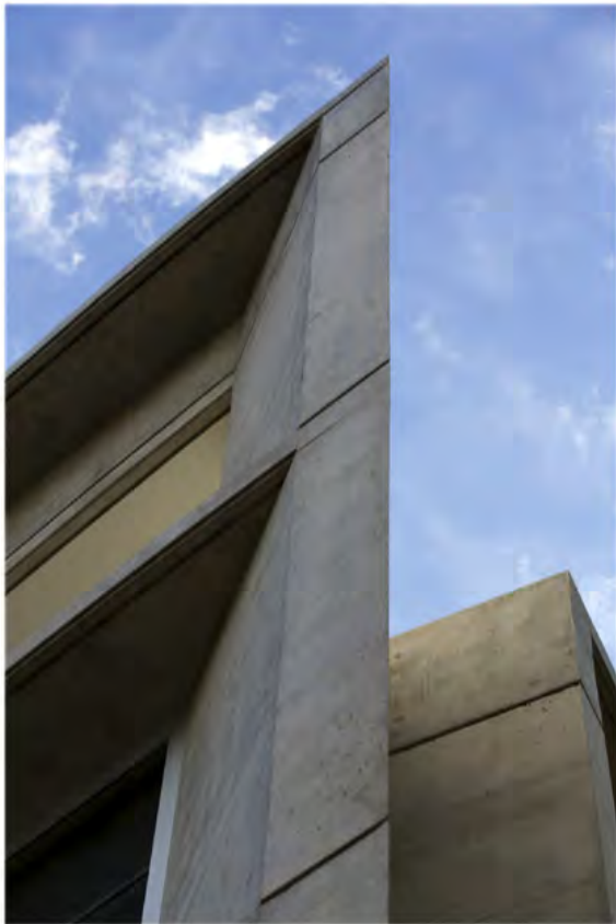
Off Form Concrete Columns
