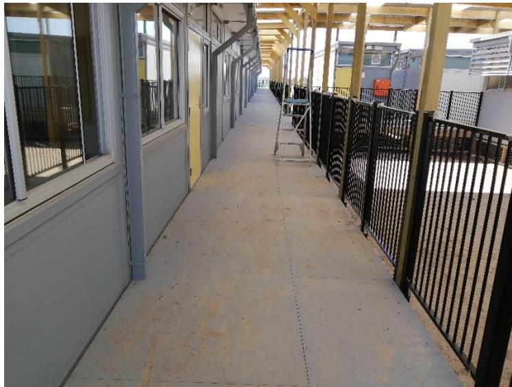
Figure 26: General photo- Timber decking
