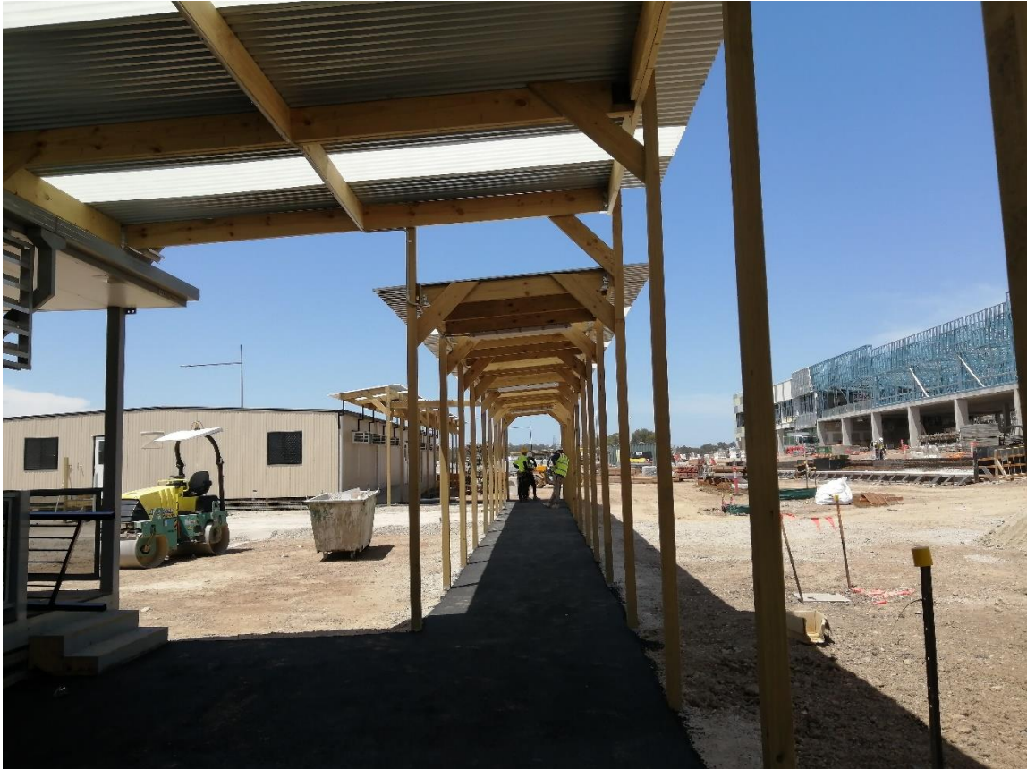
Figure 37: General photo- Lightweight awning
