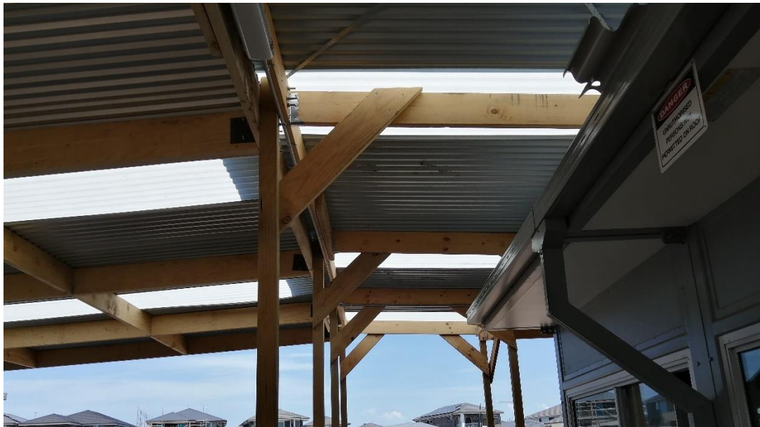
Figure 21: General photo- Awning bracing
