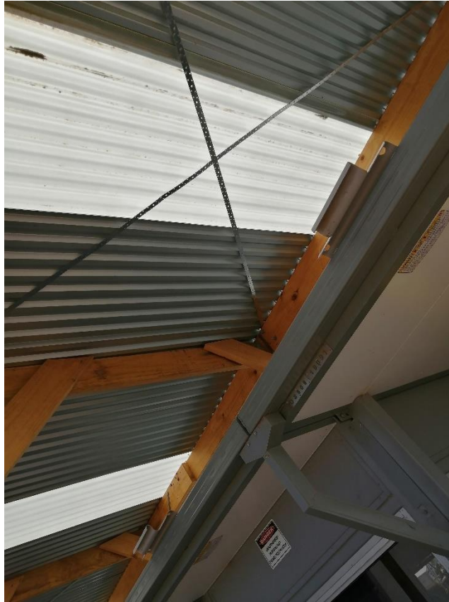
Figure 3: General photo- Awning bracing.
