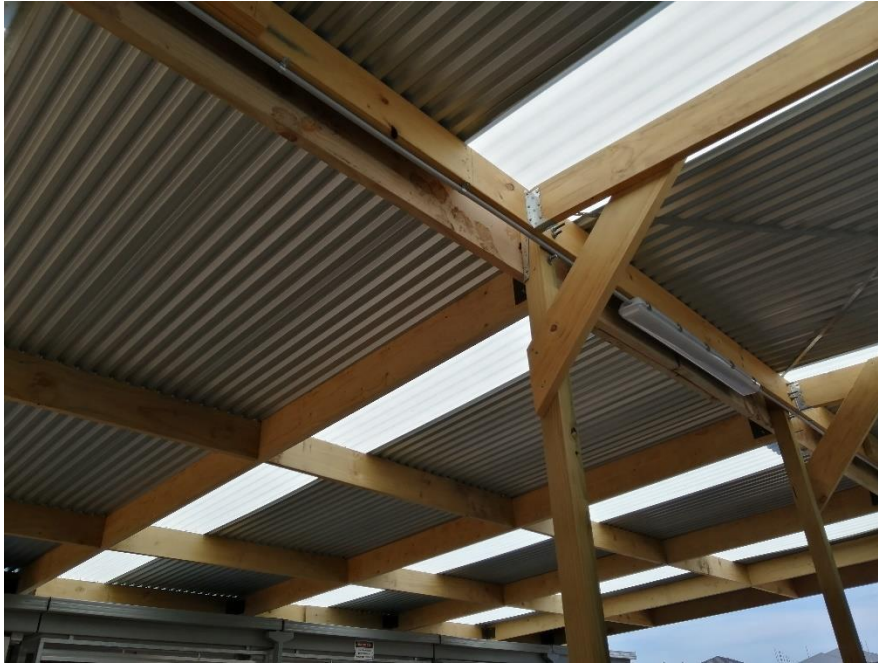
Figure 20: General photo- Awning bracing
