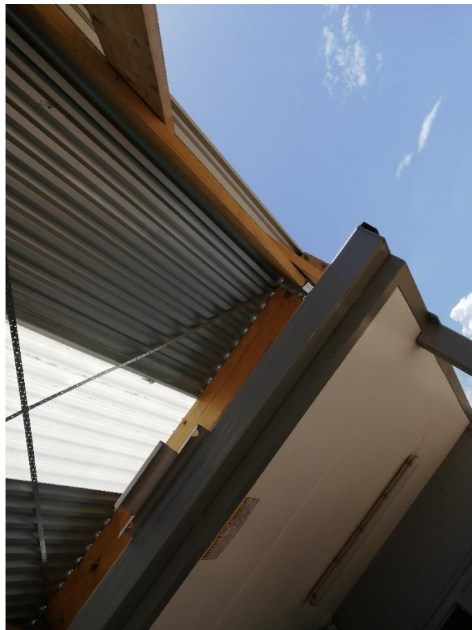
Figure 4: General photo- Awning bracing.
