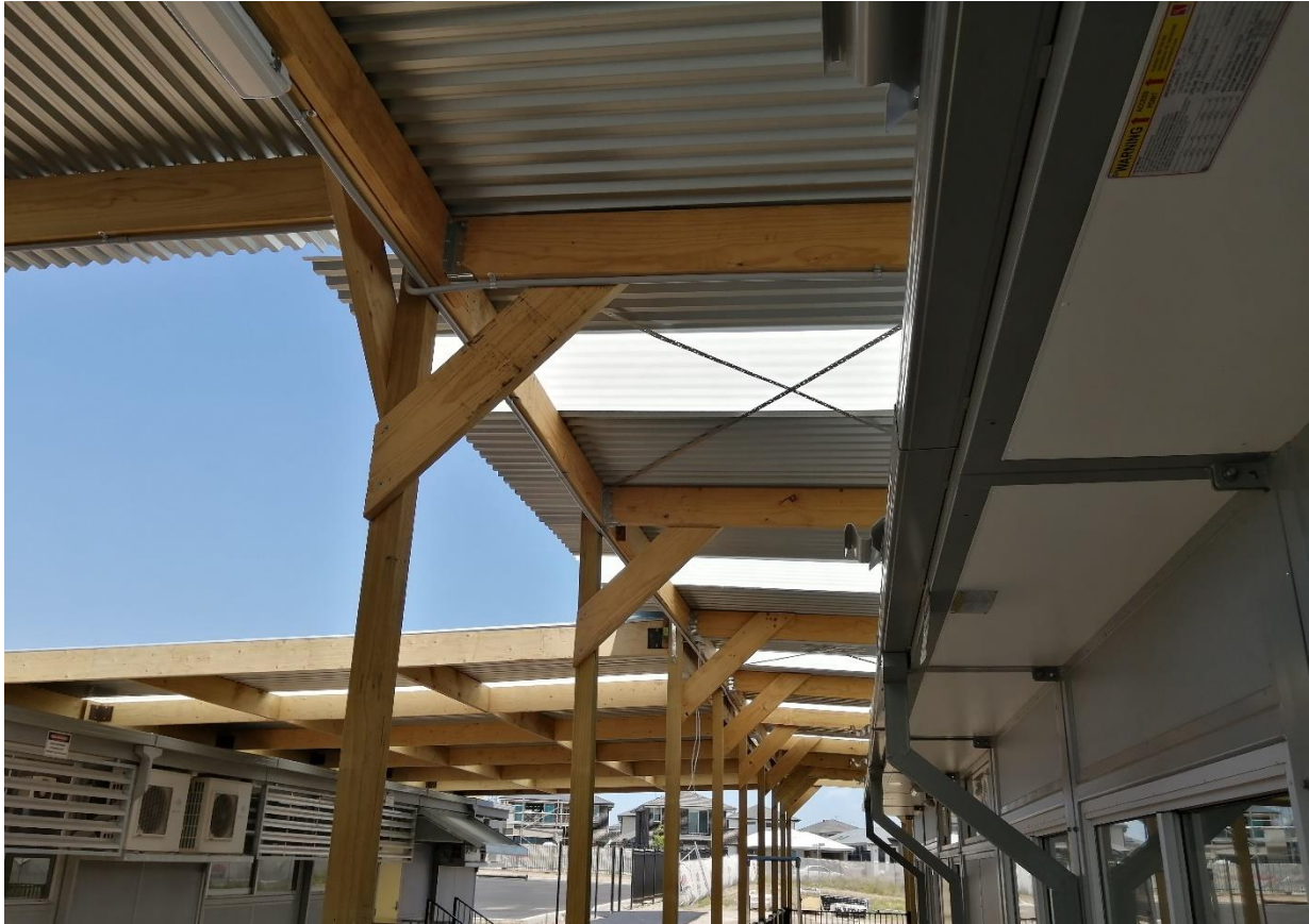
Figure 14: General photo- Lightweight awning
