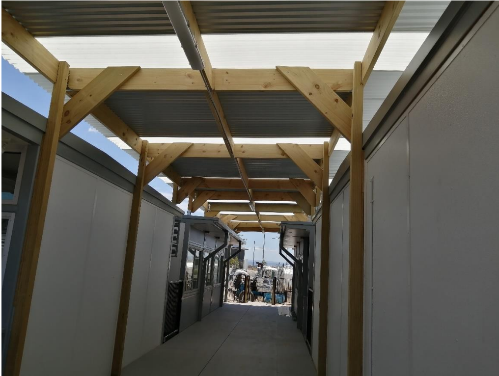
Figure 7: General photo- Lightweight awning
