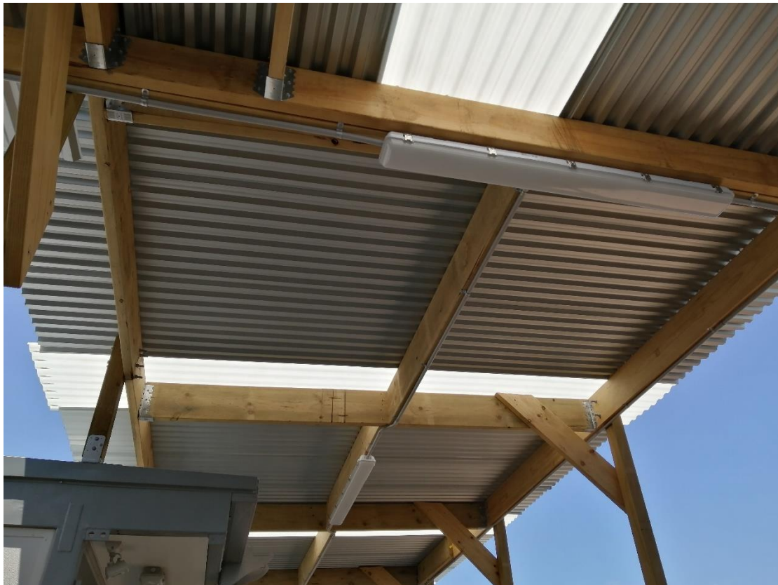
Figure 13: General photo- Lightweight awning
