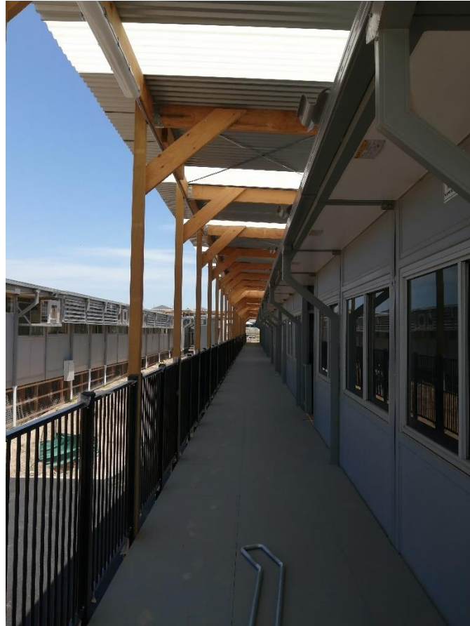
Figure 1: General photo- Lightweight awning
