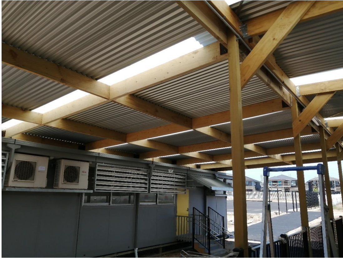
Figure 16: General photo- Lightweight awning
