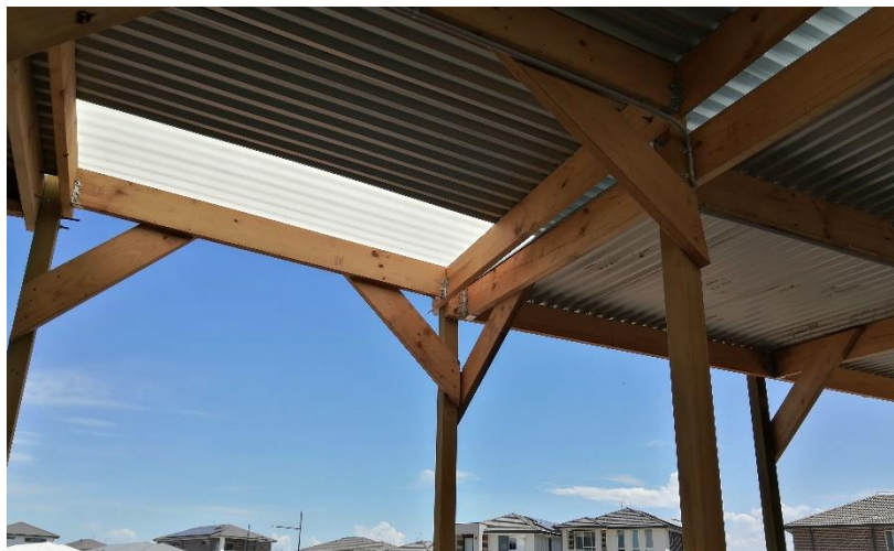
Figure 25: General photo- Awning bracing
