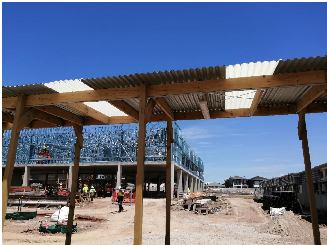
Figure 38: General photo- Lightweight awning
