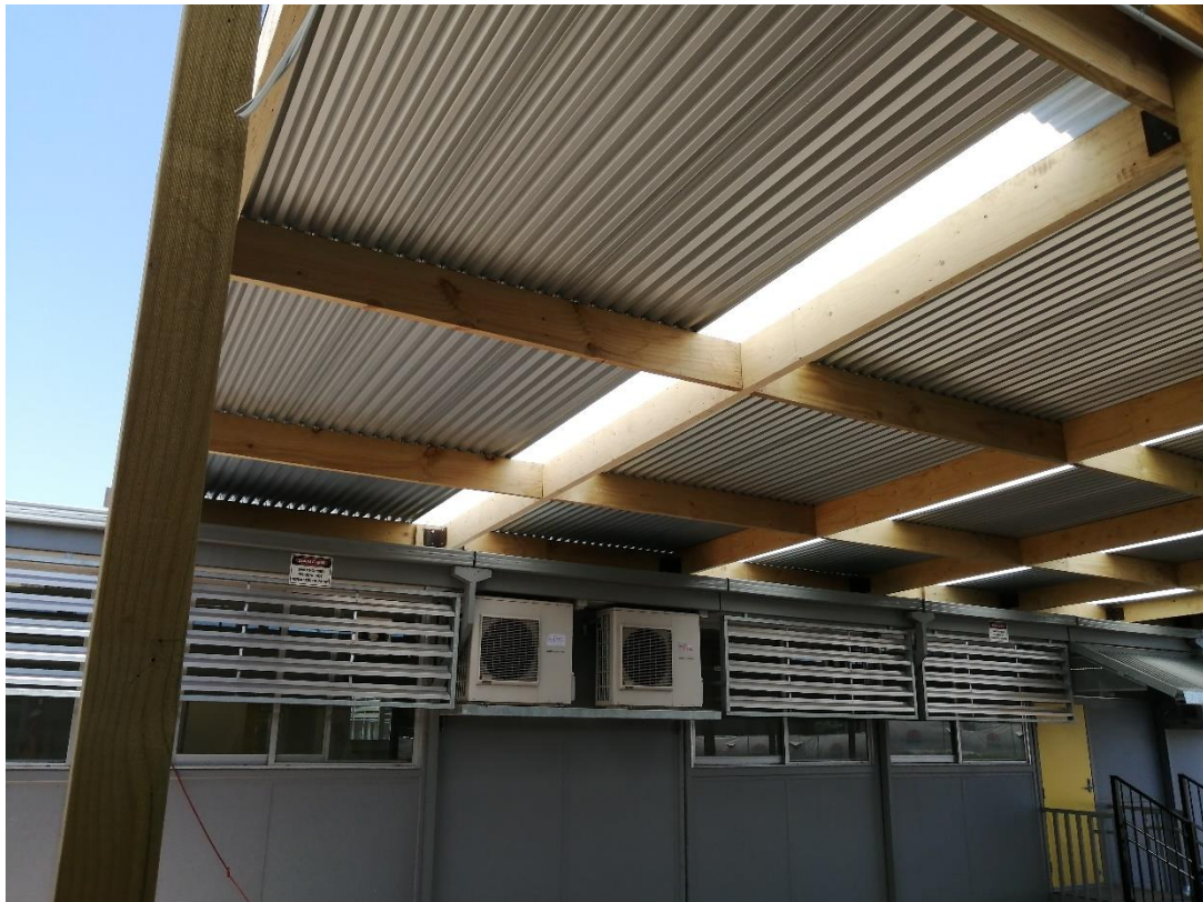
Figure 17: General photo- Lightweight awning
