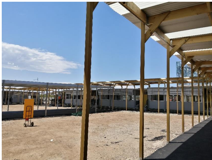
Figure 30: General photo- Timber post and awning bracing
