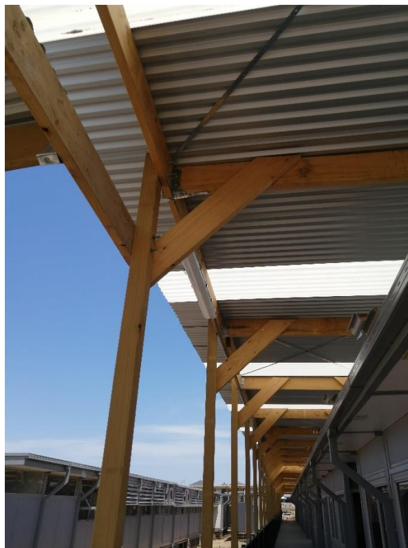
Figure 2: General photo- Lightweight awning
