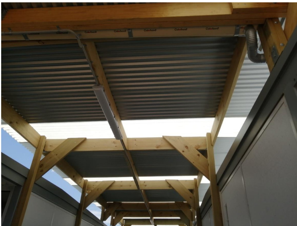
Figure 8: General photo- Lightweight awning
