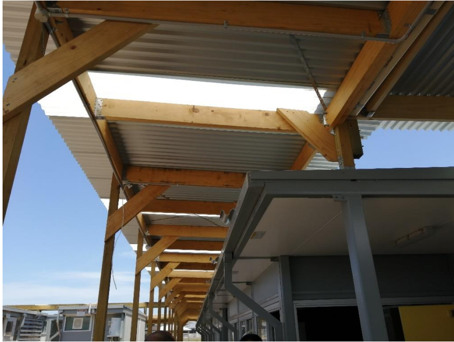
Figure 9: General photo- Lightweight awning
