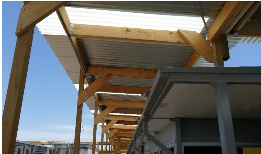
Figure 10: General photo- Lightweight awning
