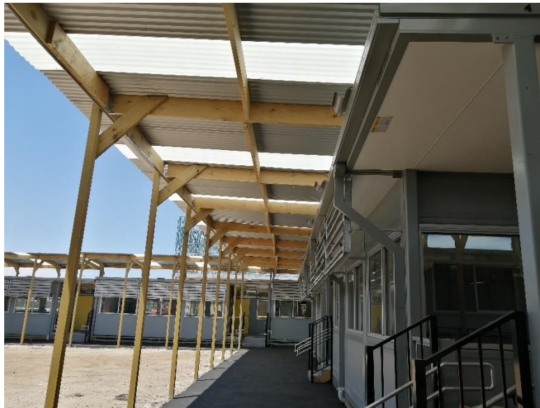
Figure 29: General photo- Lightweight awning
