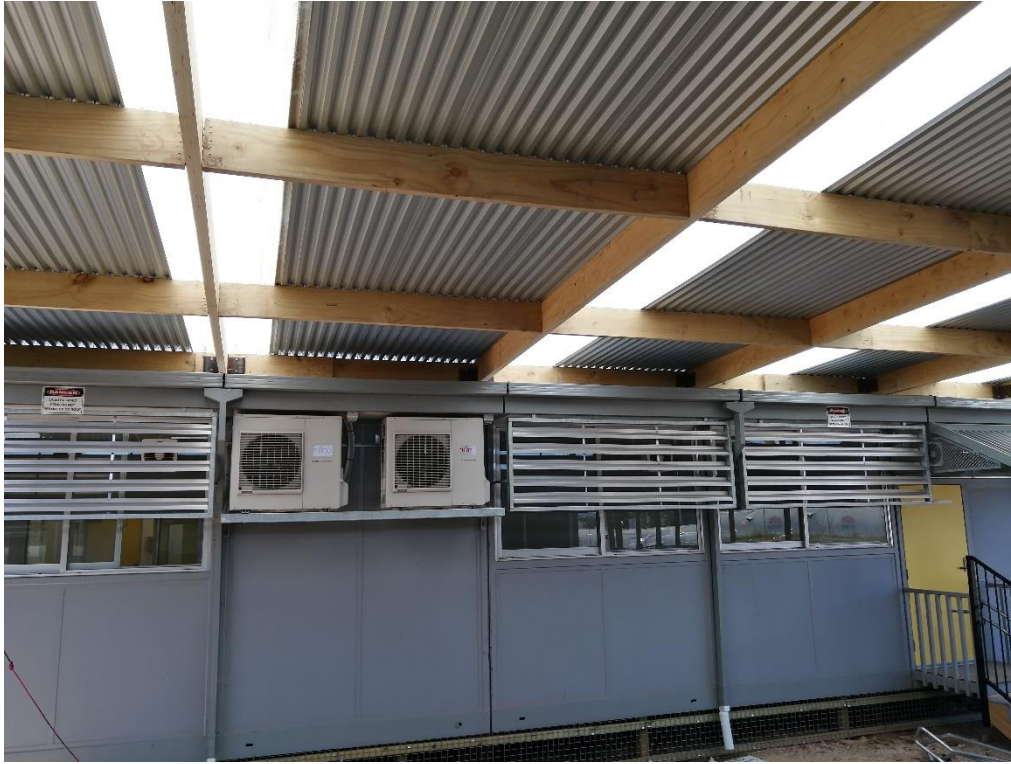
Figure 18: General photo- Lightweight awning
