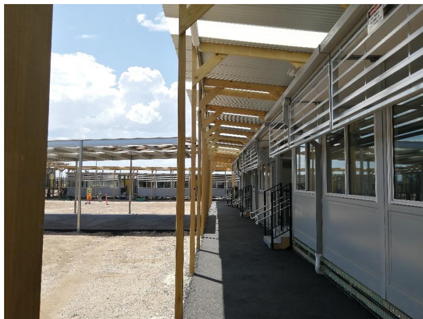
Figure 33: General photo- Lightweight awning
