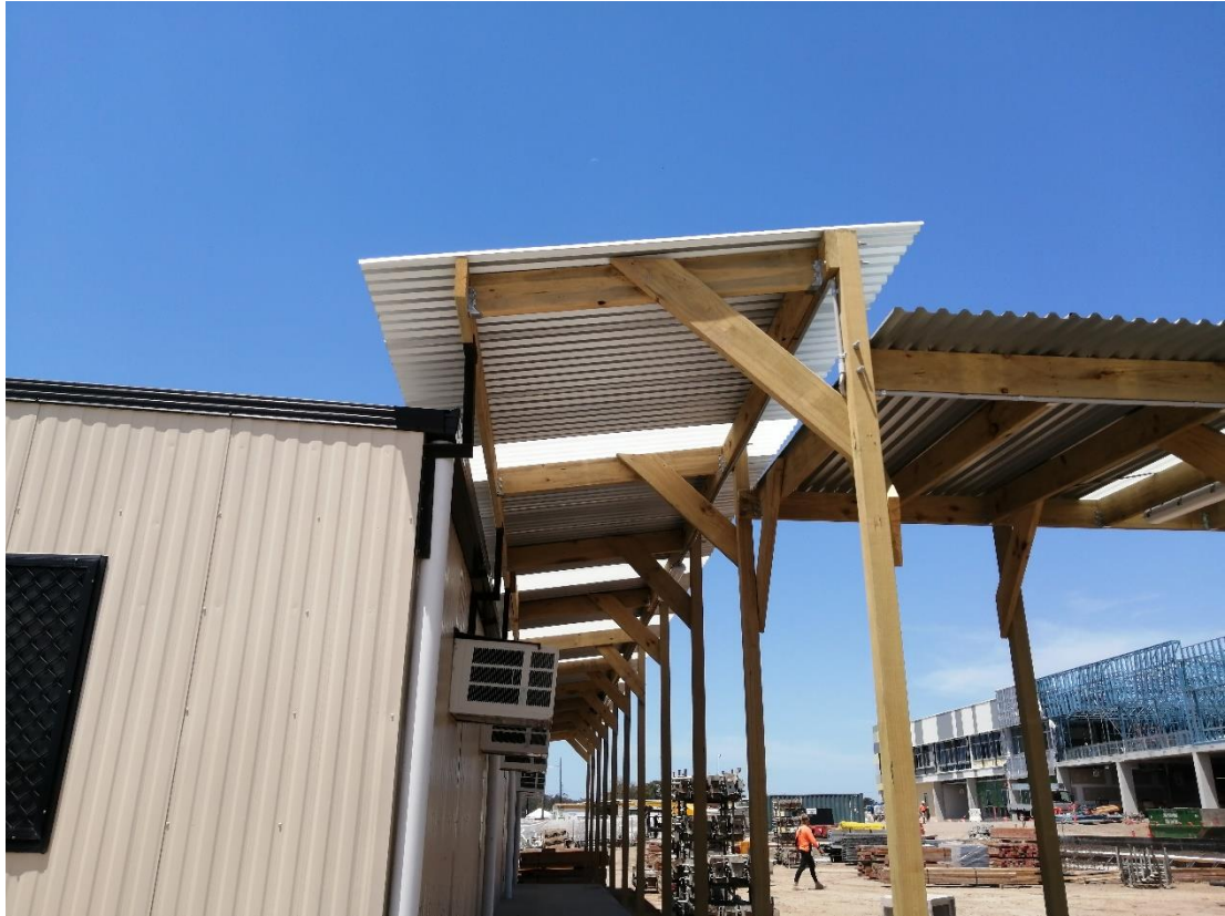
Figure 39: General photo- Lightweight awning
