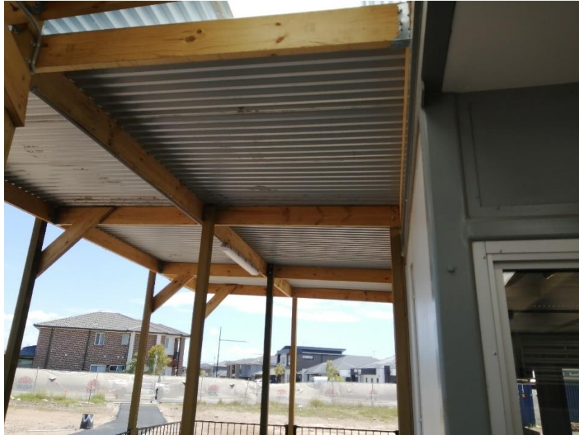
Figure 23: General photo- Lightweight awning
