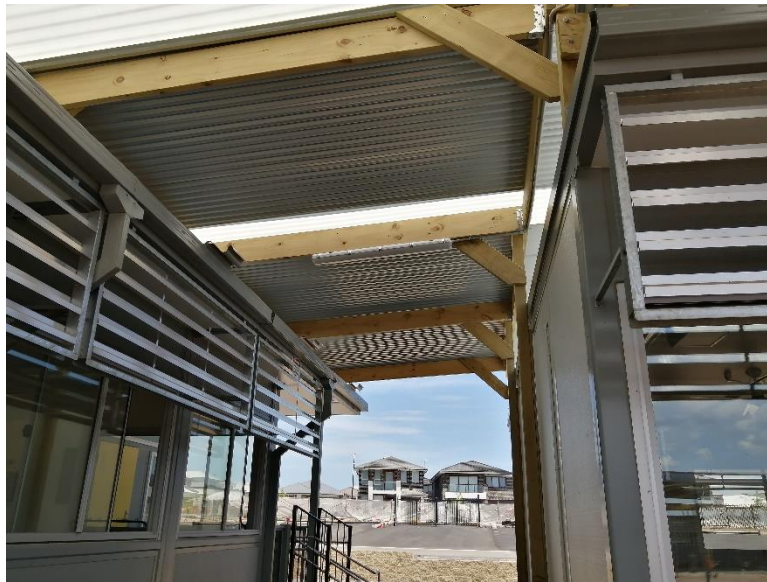
Figure 32: General photo- Lightweight awning
