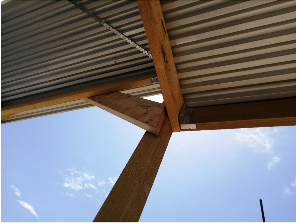
Figure 5: General photo- Awning bracing.
