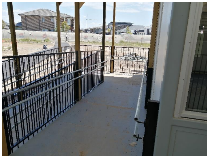
Figure 22: General photo- Ramp and handrail
