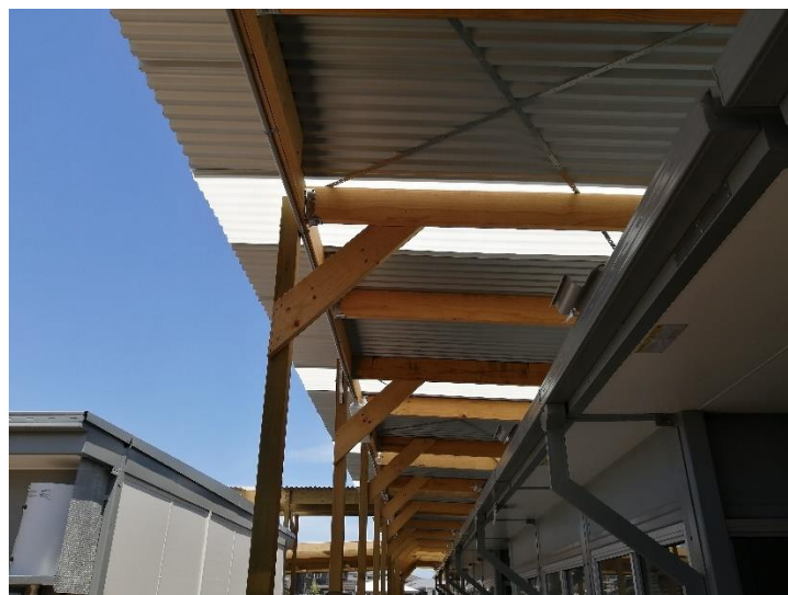
Figure 11: General photo- Awning bracing
