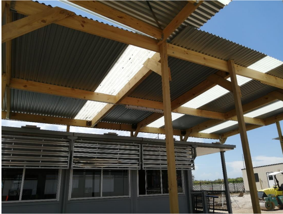
Figure 35: General photo- Lightweight awning
