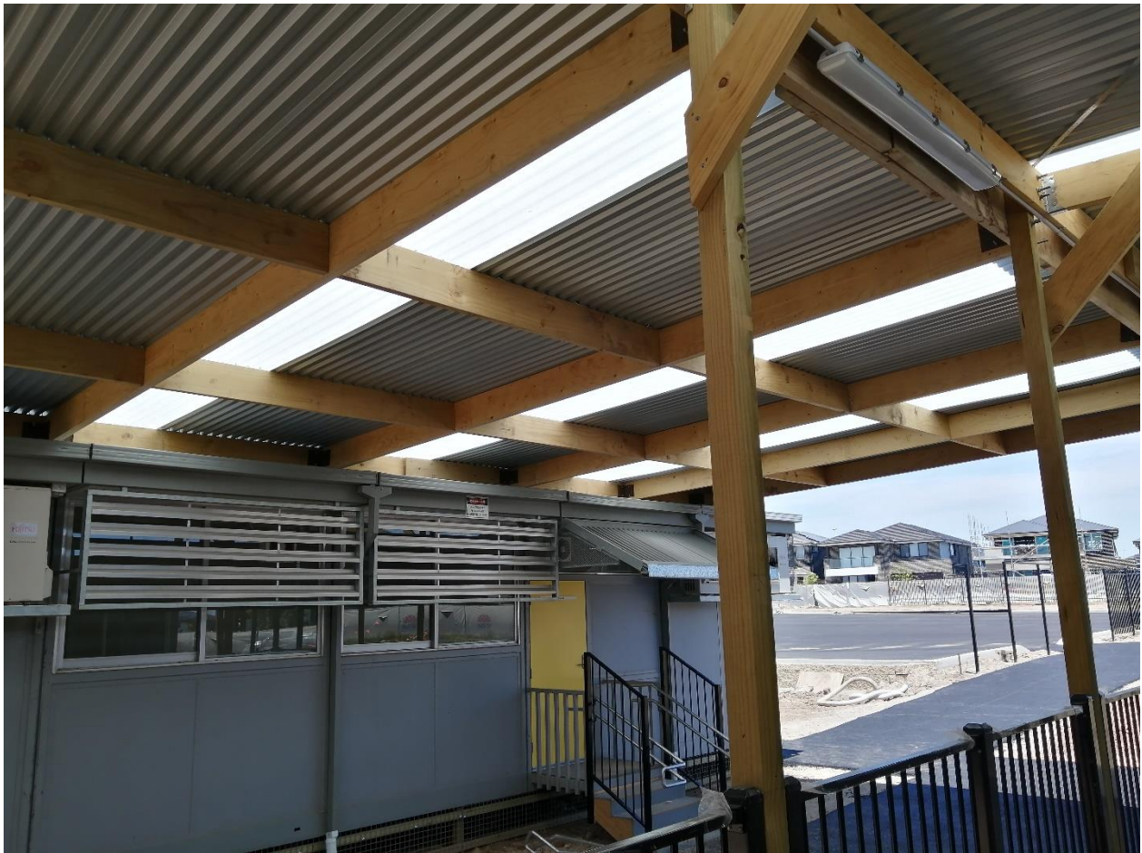
Figure 19: General photo- Lightweight awning
