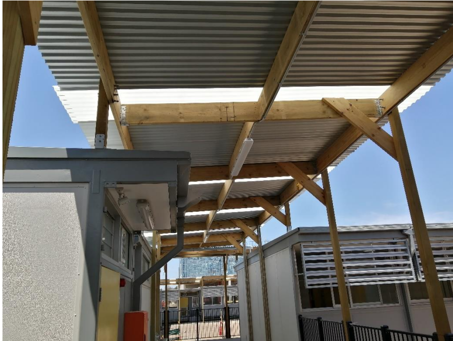
Figure 12: General photo- Lightweight awning
