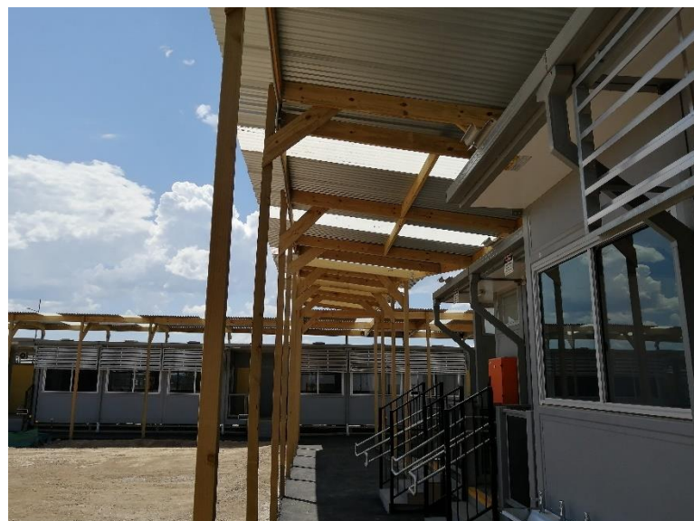
Figure 34: General photo- Lightweight awning
