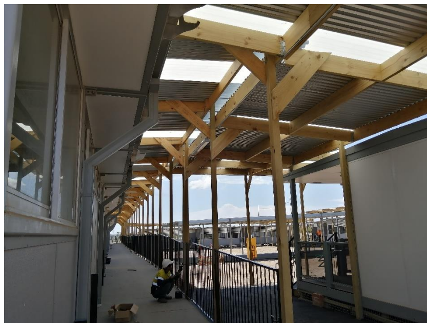
Figure 28: General photo- Lightweight awning
