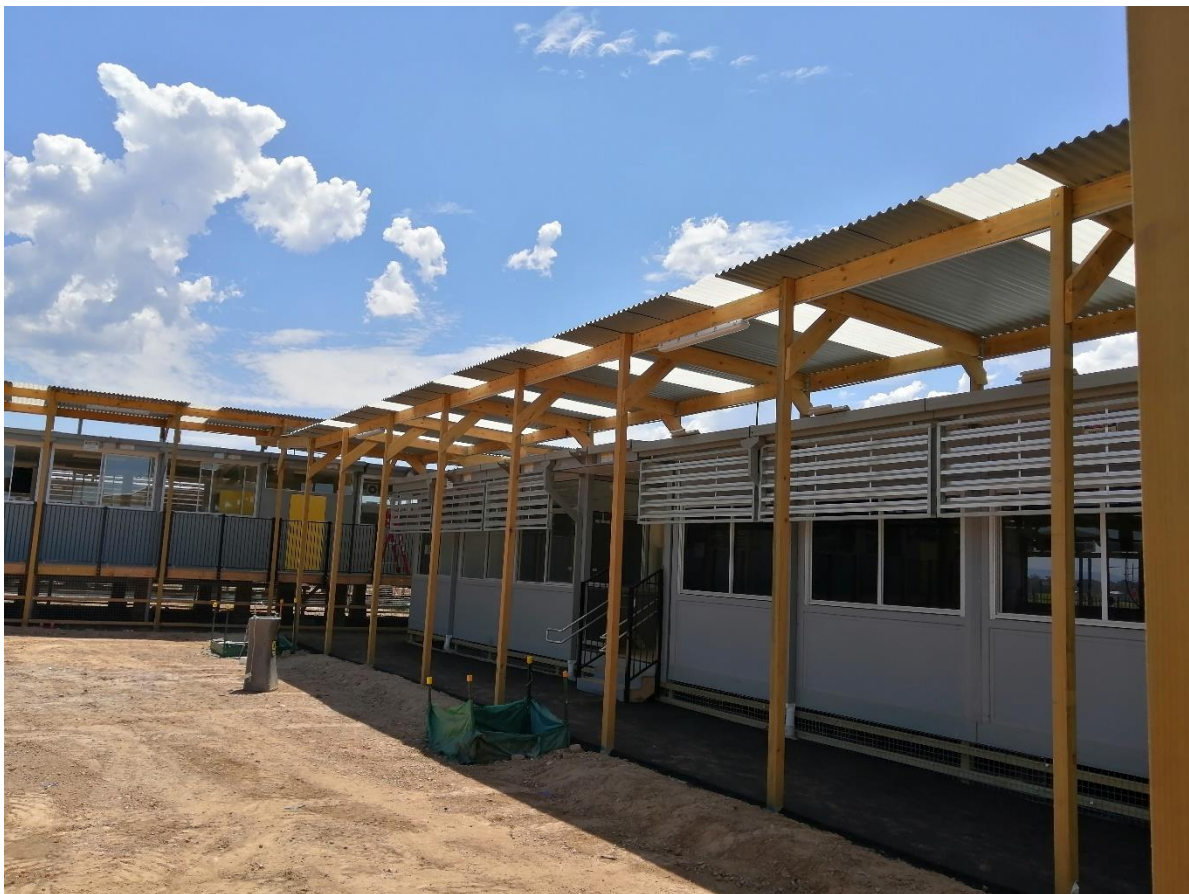
Figure 36: General photo- Lightweight awning
