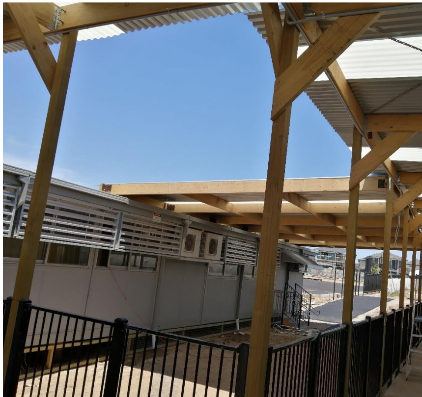
Figure 15: General photo- Awning bracing
