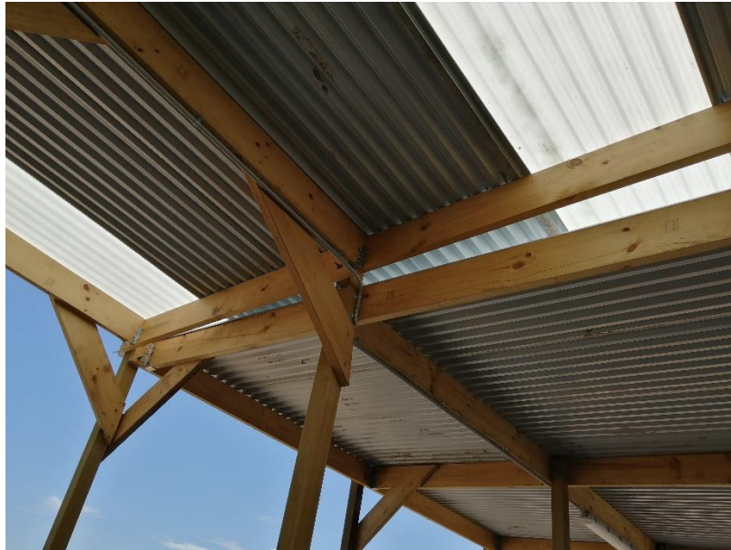
Figure 24: General photo- Awning bracing
