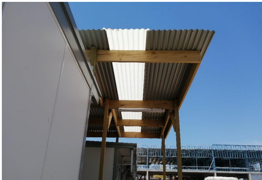
Figure 27: General photo- Lightweight awning
