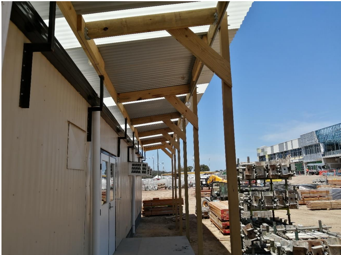
Figure 40: General photo- Lightweight awning
