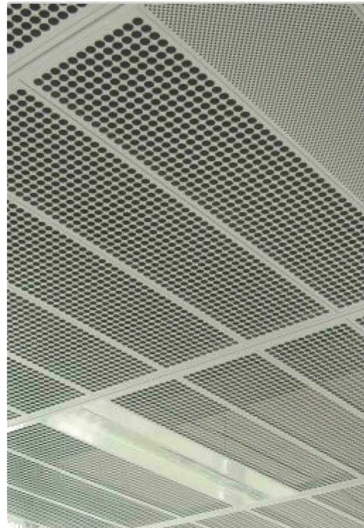
METAL PAN CEILING TO MAKER SPACES
