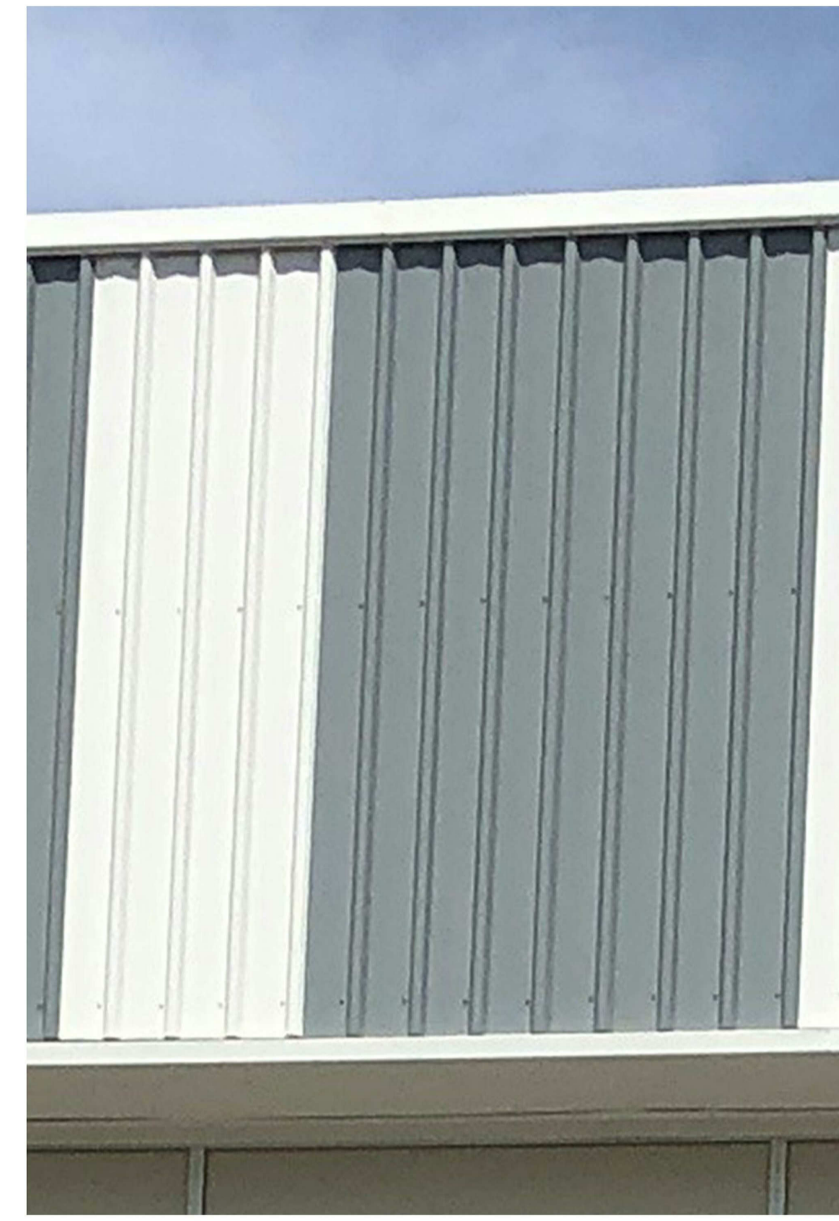
PROFILED METAL CLADDING
