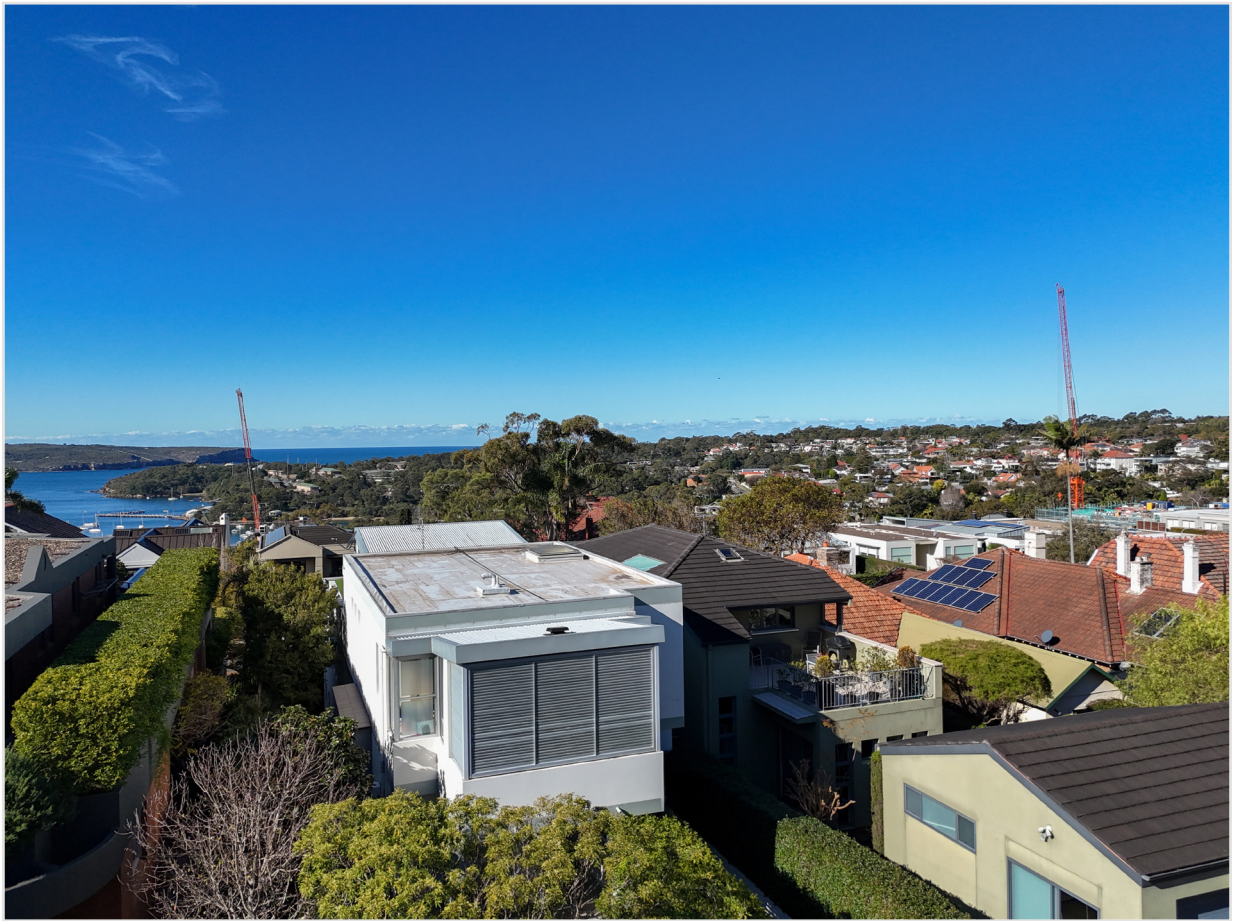
Existing site photo - Military Road (rear).
