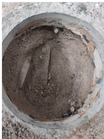
Bricks at the base of borehole
