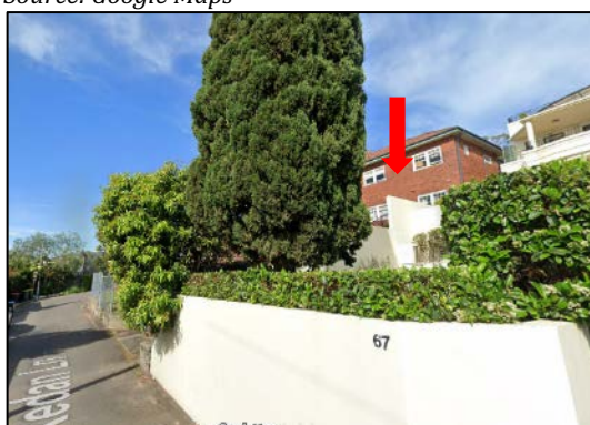
Figure 21: Oblique view towards the subject site, from Redan Lane. Source: Google Maps
