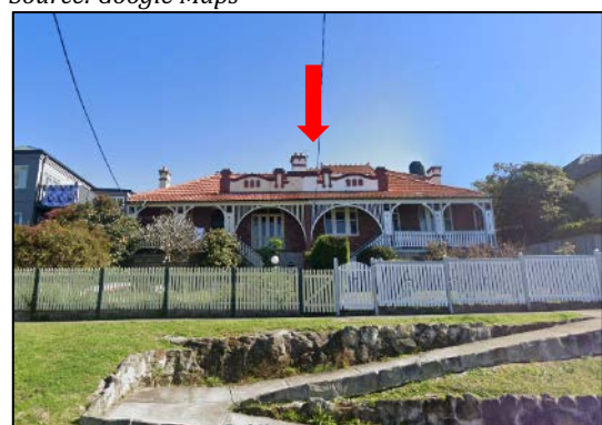
Figure 22: View from outside the heritage item at 36-38 Redan Street. The arrow indicates the location of the future development. Source: Google Maps
