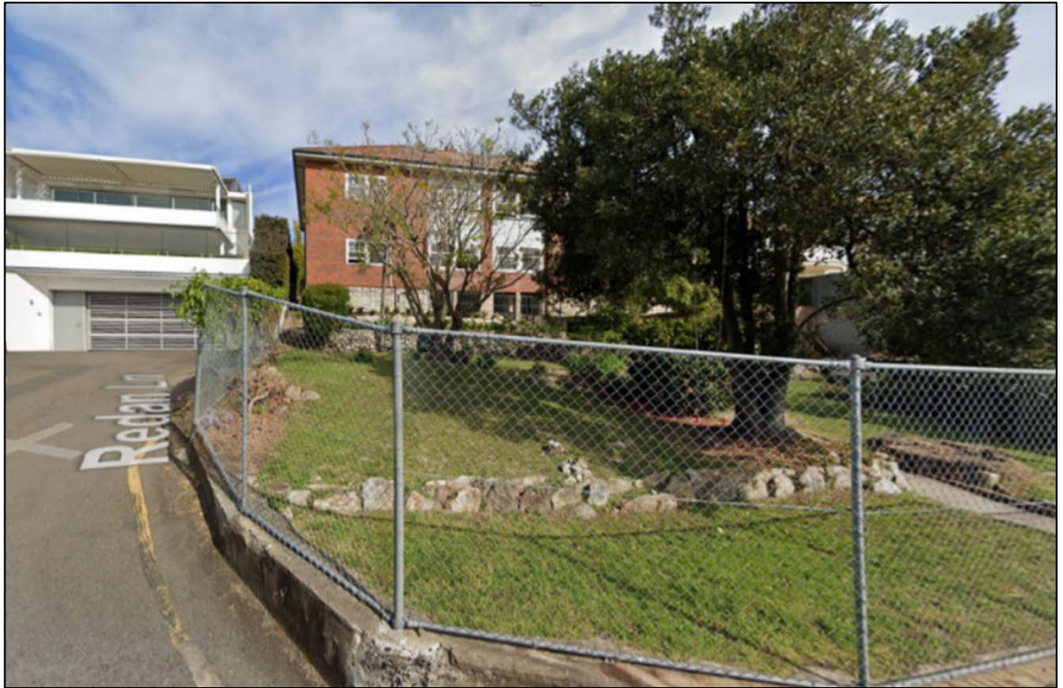
Figure 6: The site viewed from Redan Lane.
