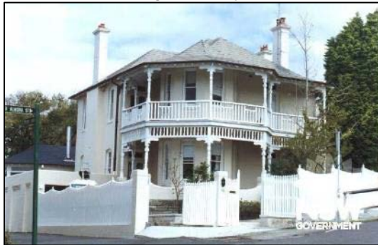
Figure 15: No. 52 Almora Street, Mosman (I13). Source: State Heritage Inventory
