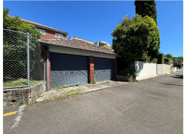
Photo 20: View north west from Redan Lane towards the rear garage on the site
