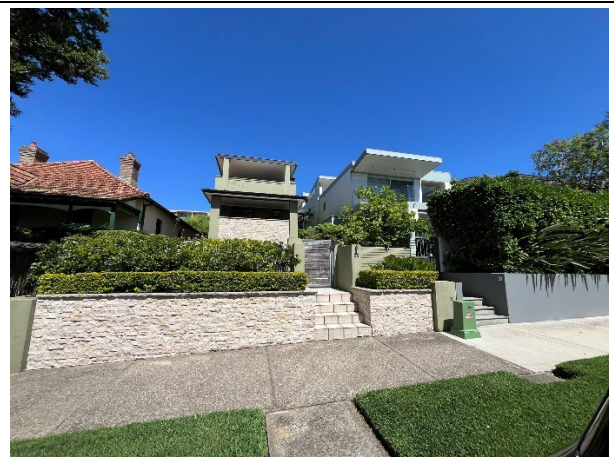
Photo 31: View looking north of, from left to right, No's 64, 66 and 68 Muston Street
