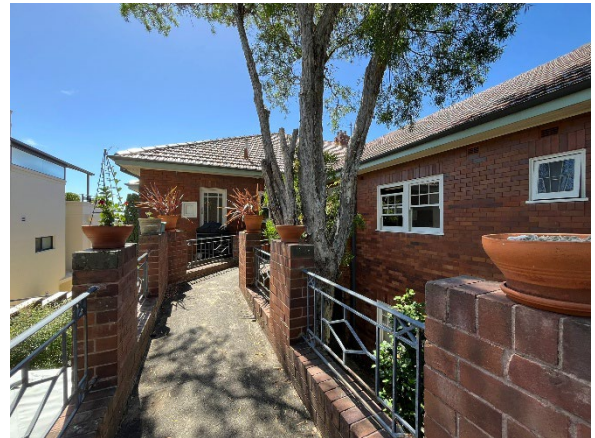
Photo 4: Elevated walkway access to upper floor units
