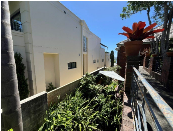
Photo 9: View east alongside setback from the northern boundary of the site with No.67 Muston Street at left and centre
