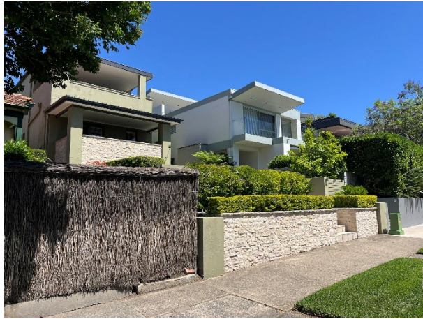
Photo 32: View looking north towards No's 66 and 68 Muston Street
