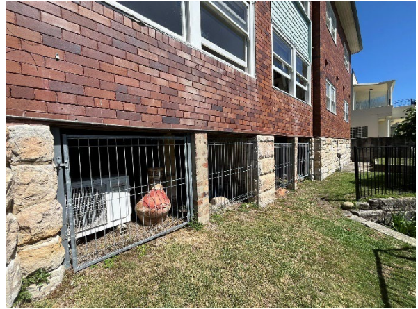
Photo 16: Sub-floor space at the rear of the existing building
