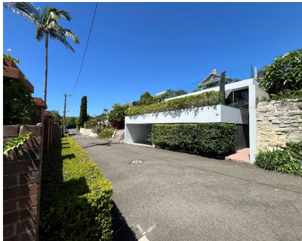
Photo 34: View to the south west along Redan Lane
