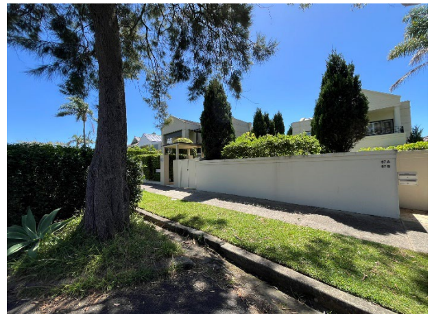
Photo 24 No. 67 and 69 Muston Street seen from Muston Street
