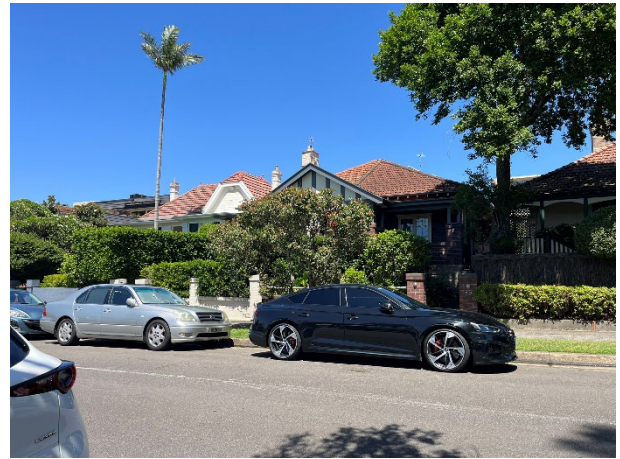
Photo 29: View looking north towards No. 60 Muston Street
