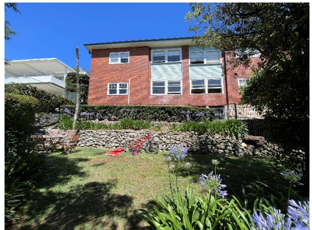
Photo 18: View looking west towards the rear of the existing building. No. 63 is at left of picture
