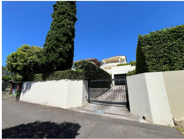
Photo 28: View of rear of No. 67 Muston Street, seen from Redan Lane. The existing building on the site is at centre left.
