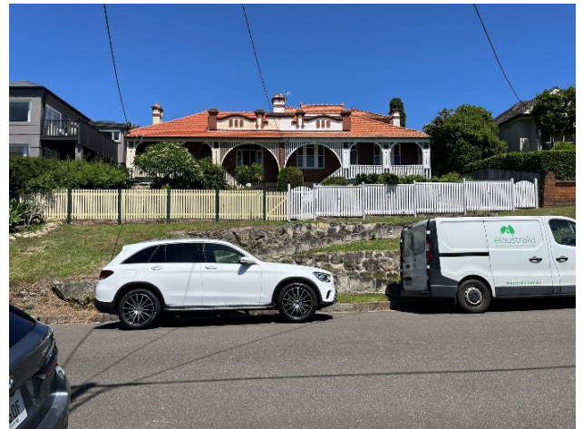
Photo 35: View of the front of the pair of heritage-listed semi-detached dwellings at No's 36 – 38 Redan Street, looking west from Redan Street
