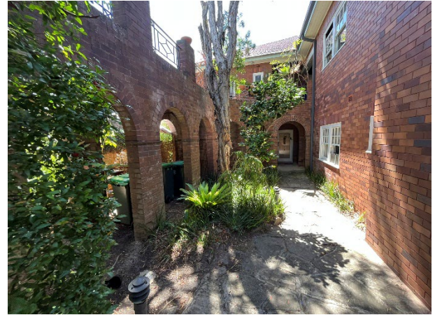
Photo 8: Northern side of existing building and elevated walkway
