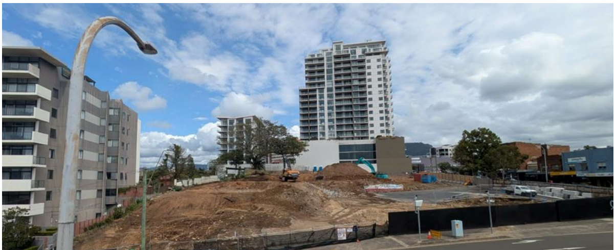
Figure 5 Photograph of site viewed from eastern side of Gladstone Avenue.
