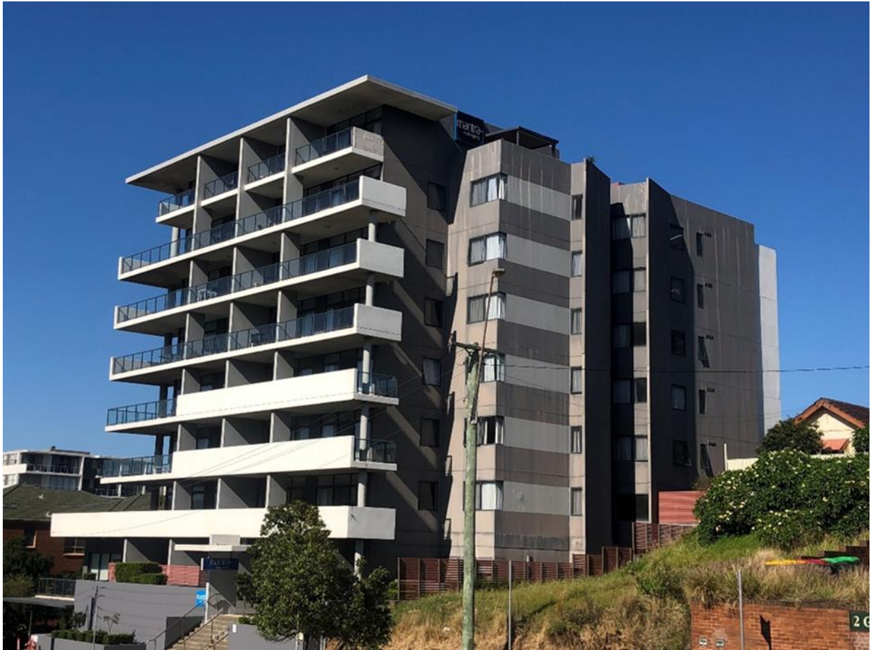
Figure 11 Photograph of the Mantra Serviced Apartments building to the south of the site
