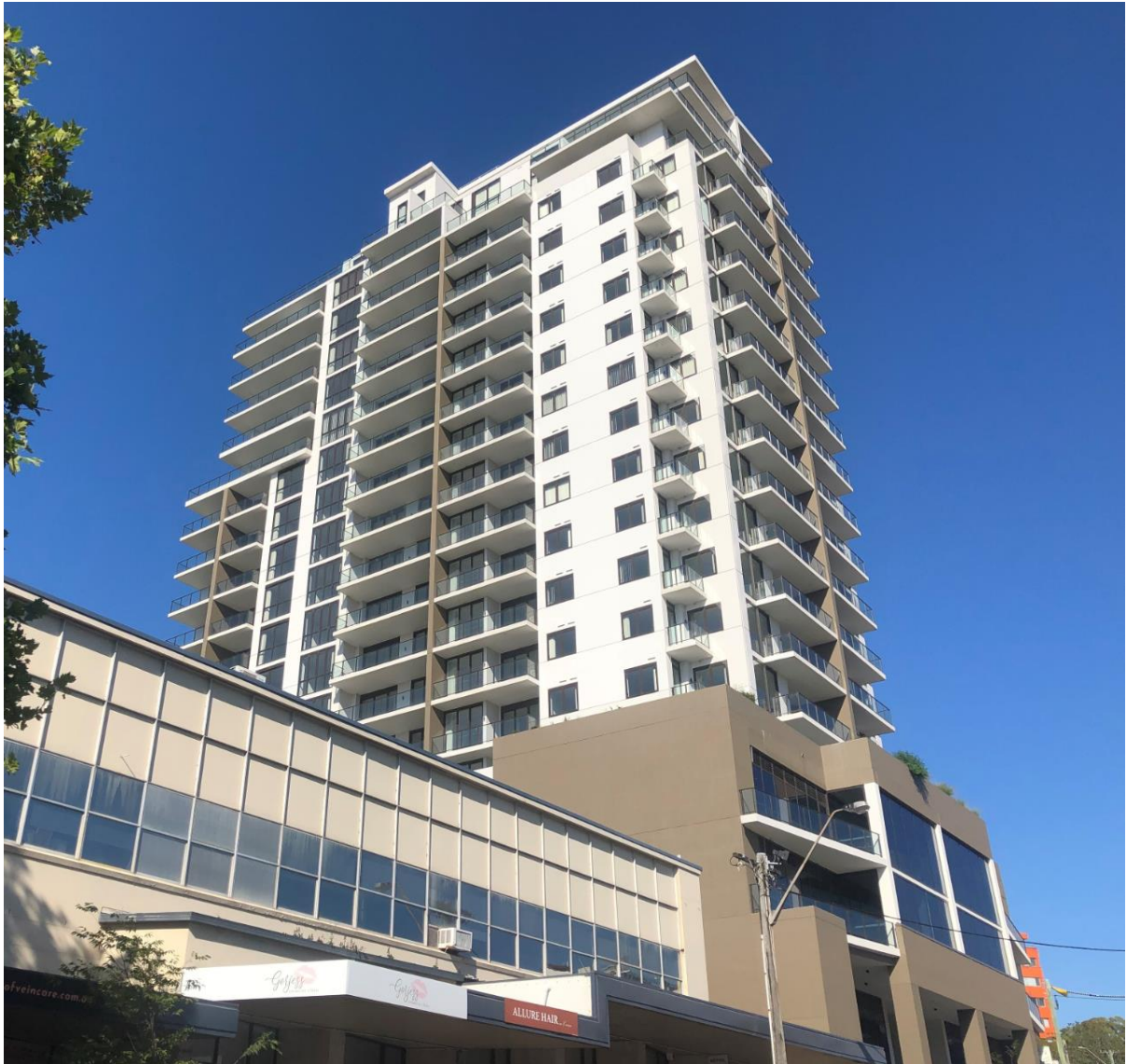
Figure 10 Completed multi-storey residential development at No 373 Crown Street, Wollongong
