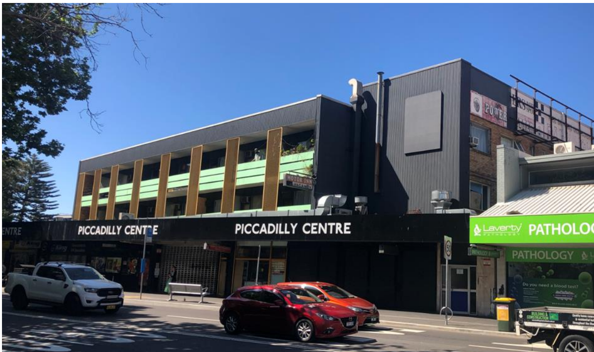
Figure 13 Photograph of the Piccadilly Centre building adjacent to the entrance to Wollongong Railway Station
