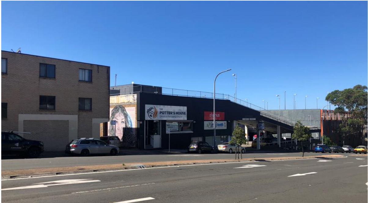
Figure 14 Photograph of the rear of Browns Corner and Piccadilly Centre viewed from Gladstone Avenue
