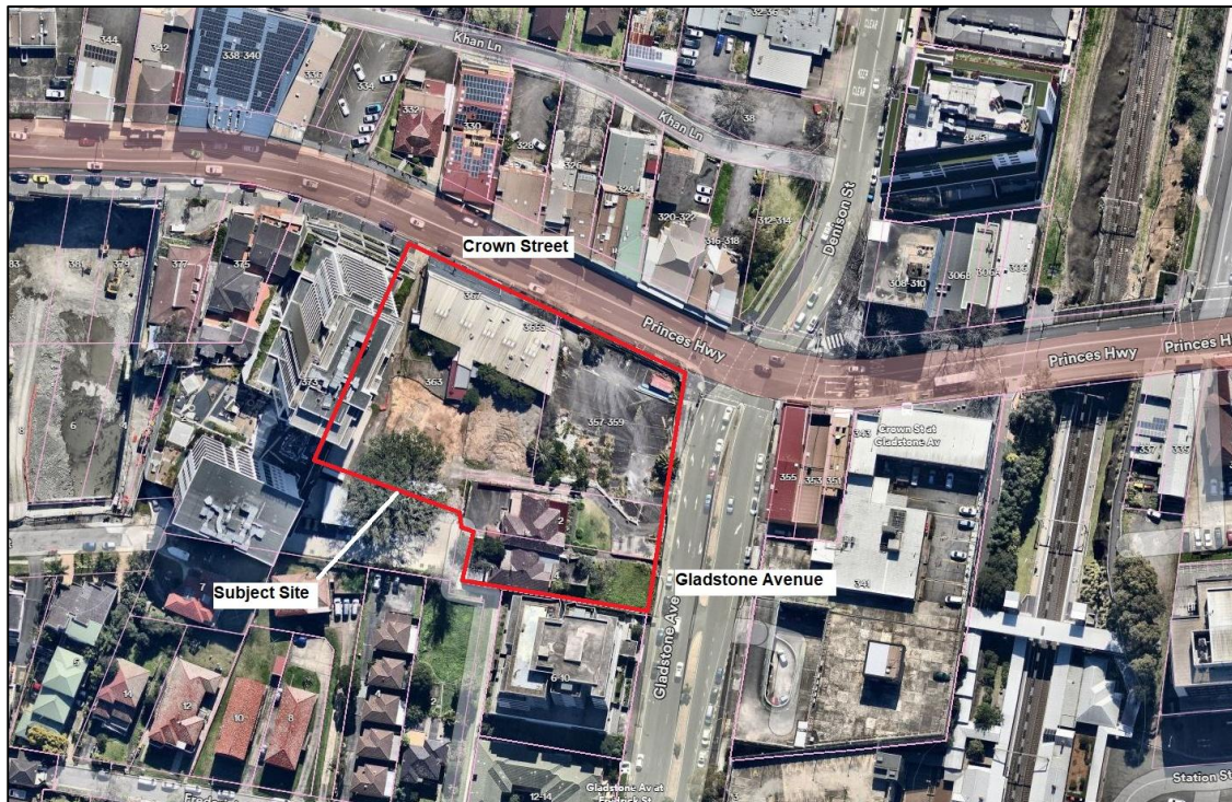
Figure 1. Aerial view of the subject site which is outlined in red (Source: Provided by Level 33 on 22 January 2026).
