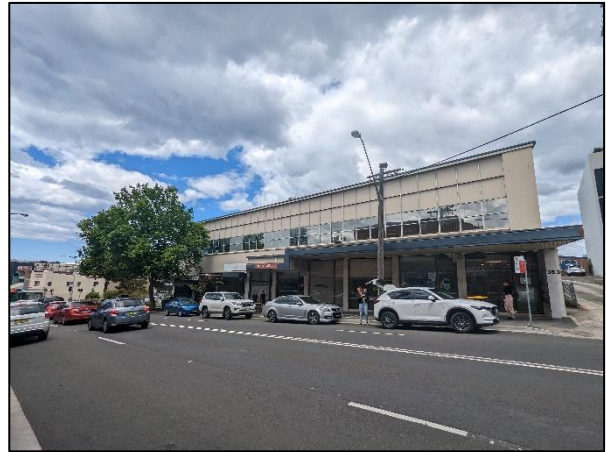
Figure 12. External view of the former two-storey mixed use building located along Crown Street.
