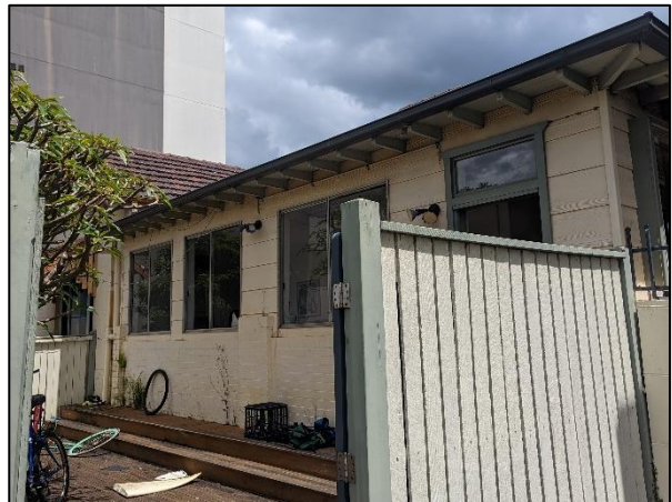
Figure 22. External front view of the former single storey dwelling at 4 Gladstone Avenue.
