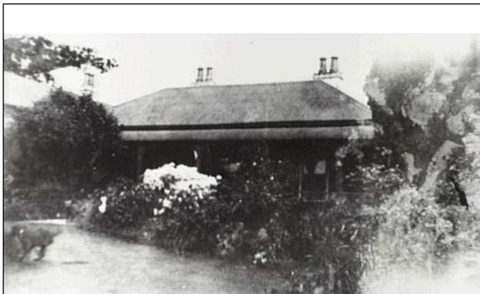
Figure 7. Undated historical photograph of Gladstone House (Source: Image number: P08/P08319, Wollongong City Libraries).
