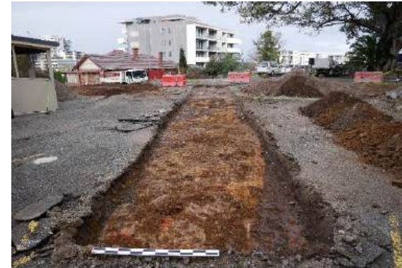
Figure 17: Showing 018 facing south
