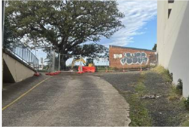
Figure 2: Image from the entrance to the site showing cordoned off areas around the archaeological resources
