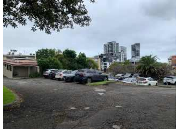
Plate 6: showing the two stepped carparks at the rear of the commercial building
