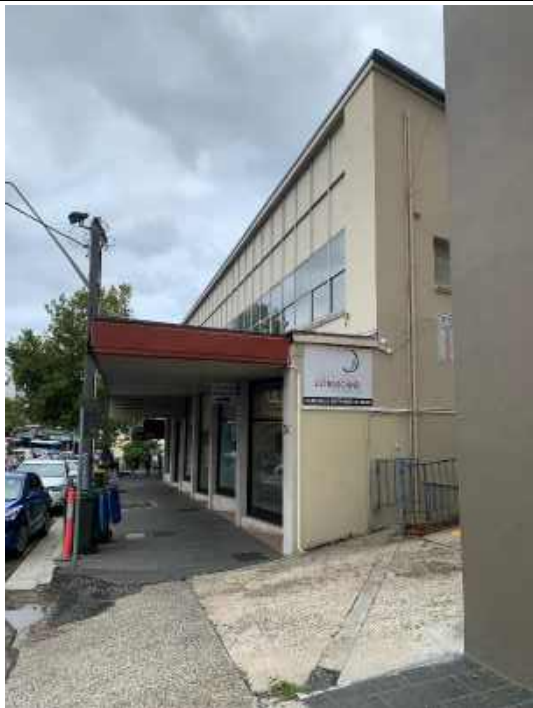
Plate 3: view of the existing commercial building
