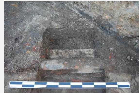
Figure 21: Showing 023 and 020 and 022. Shown is the iron capping of 020 and the internal mortar covering of the lower course of brick
