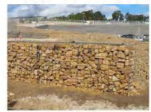
Rigid stainless steel gabion cage with 75-150mm sandstone spall 1000mm wide tree pits with weathering steel
