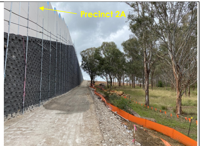
Photo 2: Looking south along the western boundary of precinct 2A. Photo shows the perimeter sealed maintenance track, sound barrier and retaining wall.
