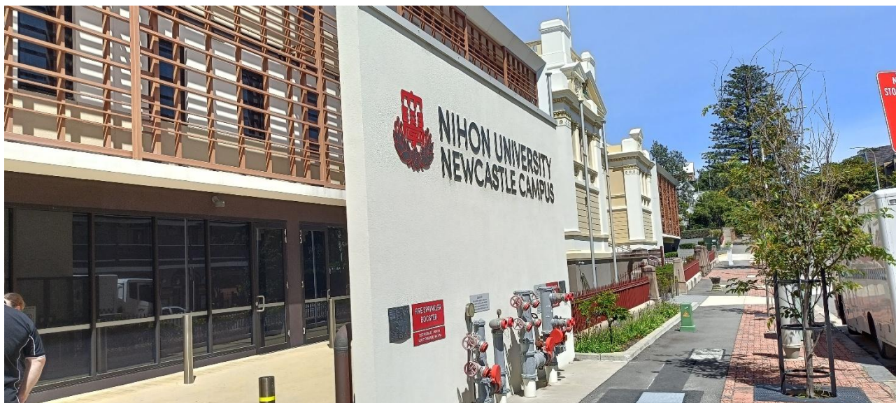
Photograph 2.1 View of the property looking west on Church Street
