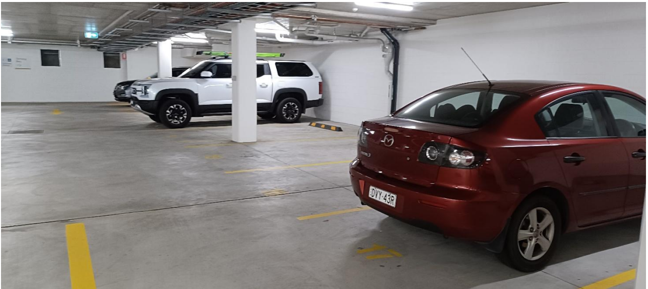
Photograph C.5 Carparking area in underground carpark
