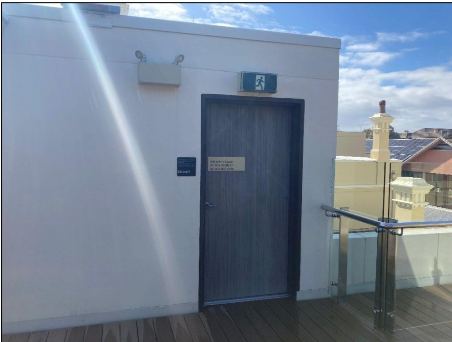
Figure 11 – Rooftop emergency exit
