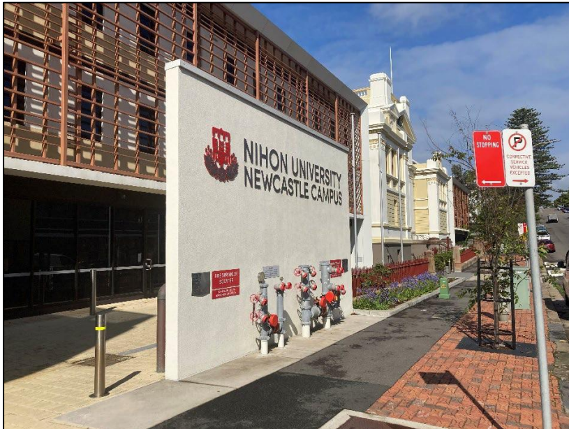
Figure 2 – General external photo of building
