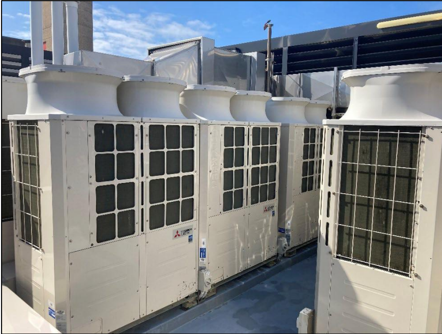
Figure 12 – Rooftop HVAC area
