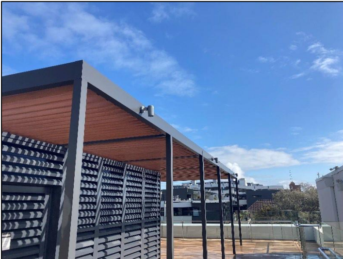
Figure 13 – Exterior of rooftop HVAC area, noting downward facing lights
