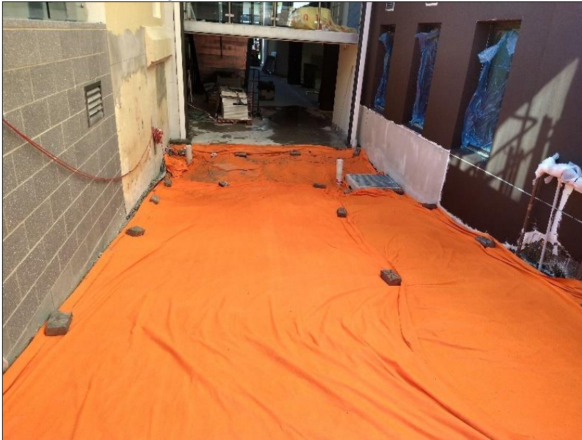
Figure 23 – Orange geofabric marker layer in garden bed at the rear of the Atrium (16 July 2021)
