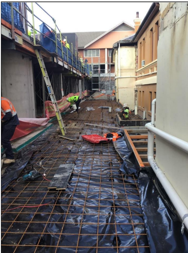
Figure 26 - Black plastic marker layer beneath Atrium concrete slab (25 August 2020 - supplied by Built)
