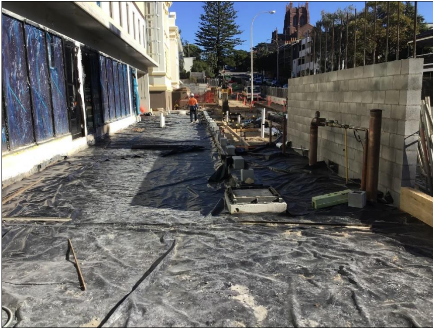
Figure 27 – Black plastic marker layer beneath concrete pavement on northern (front) side of Student Accommodation Building (26 June 2021 – supplied by Built)
