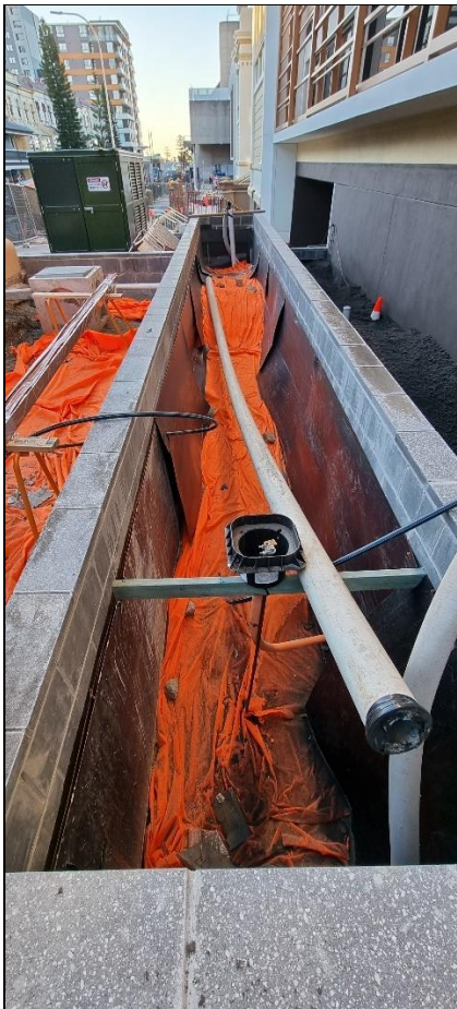
Figure 26 – Orange geofabric marker layer within garden bed/planter box on northern side (front) of the Education Building (4 August 2021 – supplied by Built)
