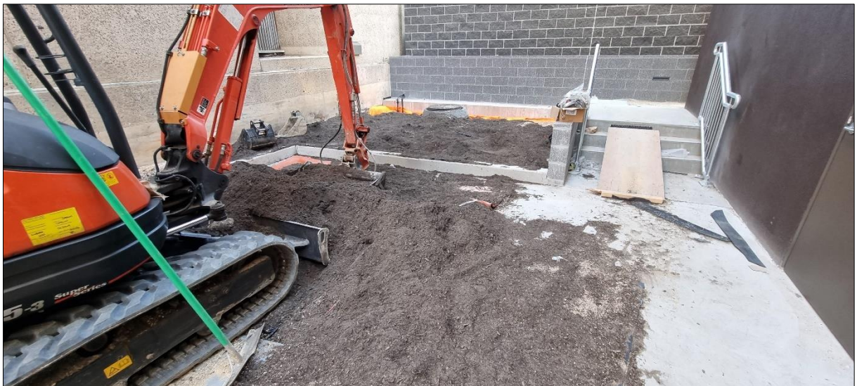
Figure 34 – Hills Premium Garden Mix used over geofab in garden beds in south east corner of site (17 August 2021 – supplied by Built)
