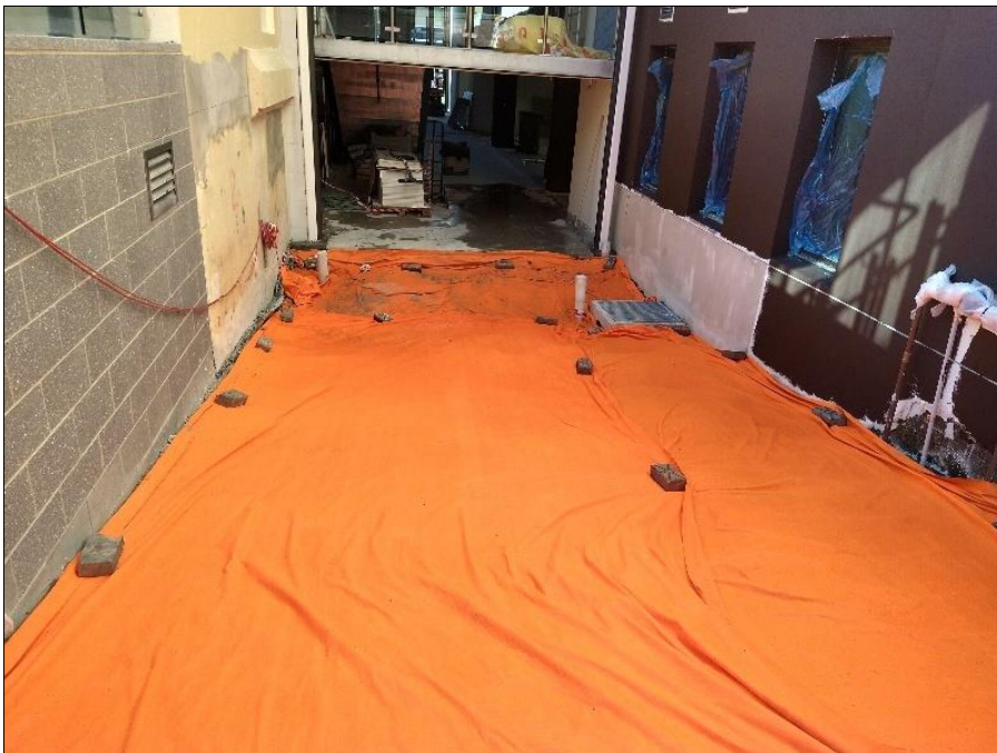
Figure 22 – Orange geofabric marker layer in garden bed at the rear of the Atrium (16 July 2021)
