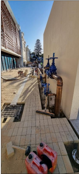
Figure 31 – Pavers laid over packing sand (from Saddingtons) over concrete (28 July 2021 – supplied by Built).
