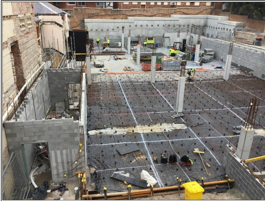
Figure 8 - Black plastic marker layer beneath Education Building concrete slab (21 September 2020 - supplied by Built)
