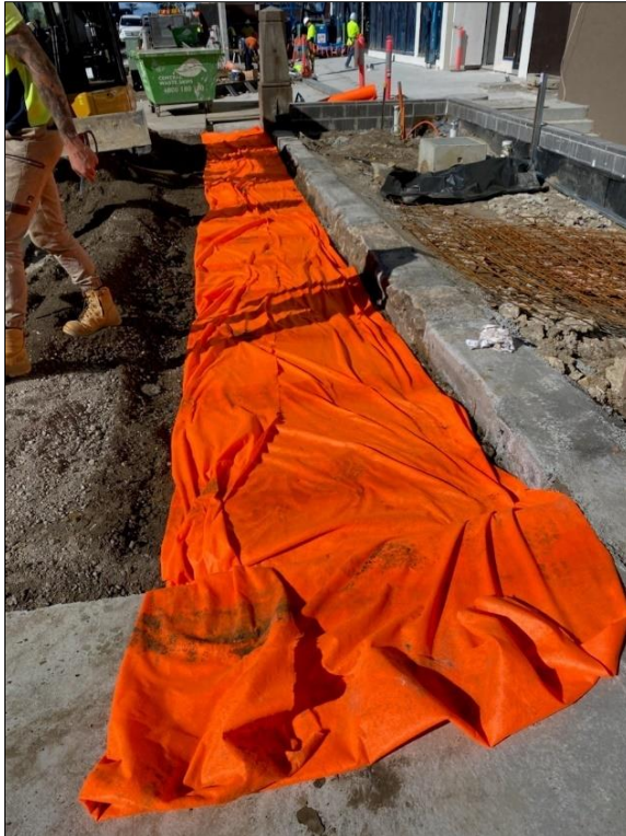
Figure 23 – Orange geofabric marker layer beneath the asphalt pavement along northern (front) boundary adjacent to footpath (19 July 2021 – supplied by Built)
