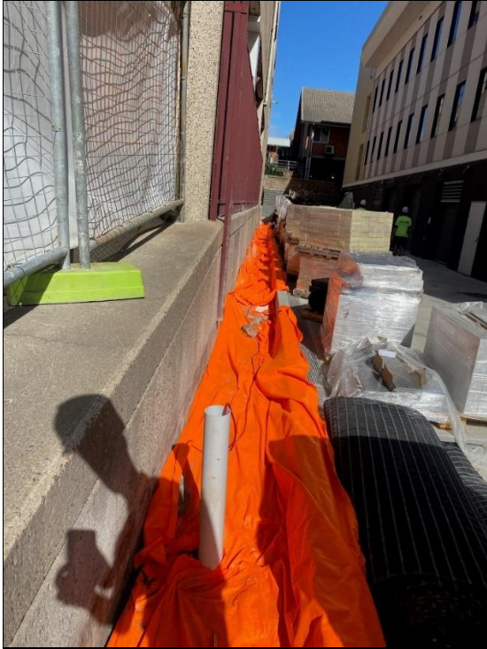
Figure 27 – Orange geofabric marker layer within garden bed/planter box on eastern side of the Student Accommodation Building (26 July 2021 – supplied by Built)
