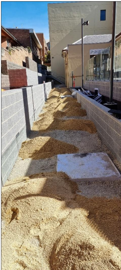
Figure 30 - Crushed granite (white Scorria) supplied by Saddingtons and Blue Gum Landscaping Centre (from Coastal Quarry Products) in process of being laid on footpath over roadbase (27 July 2021 -supplied by Built)
