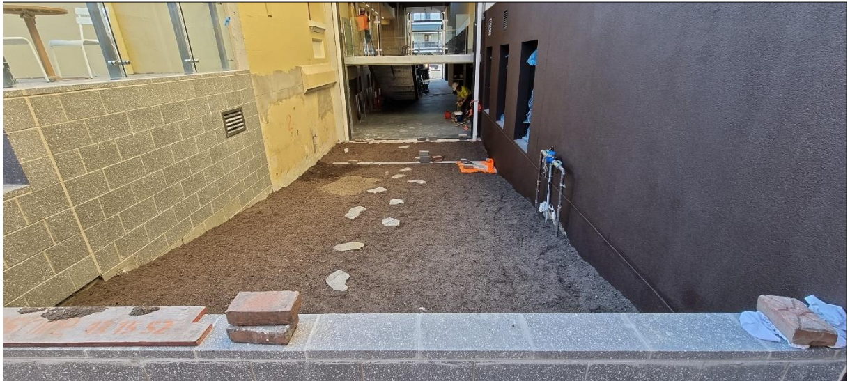
Figure 35 – Hills Premium Garden Mix used over geofab in garden beds (17 August 2021 – supplied by Built)
