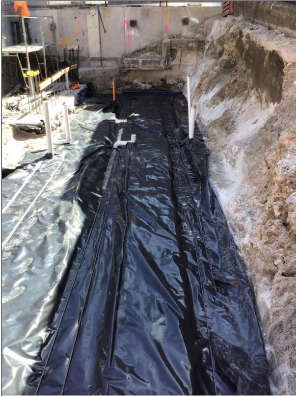
Figure 6 - Black plastic marker layer beneath concrete slab in north-west corner site (1 September 2020 - supplied by Built)
