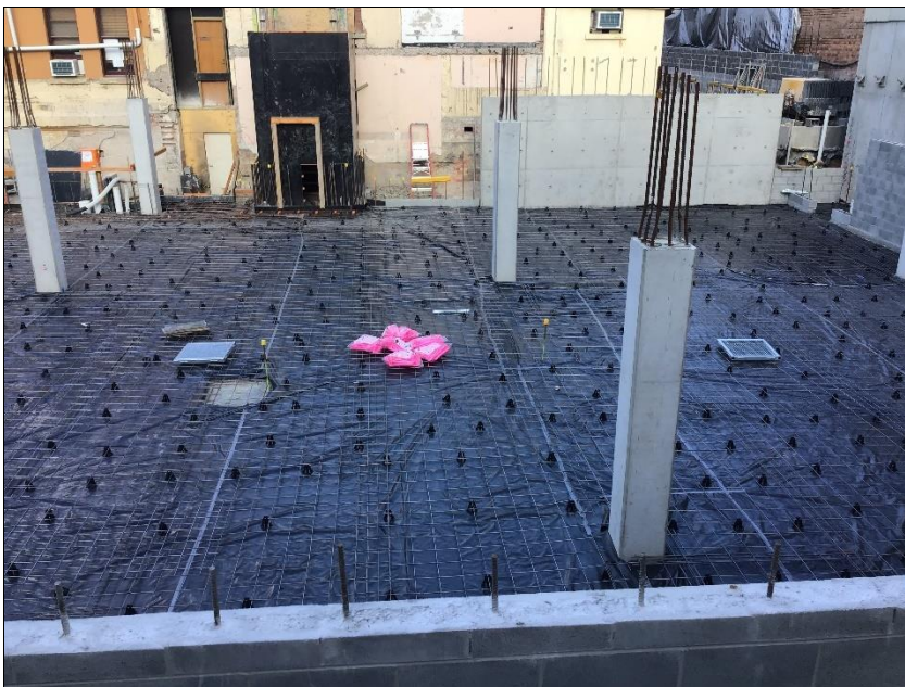
Figure 7 - Black plastic marker layer beneath Education Building concrete slab (16 September 2020 - supplied by Built)
