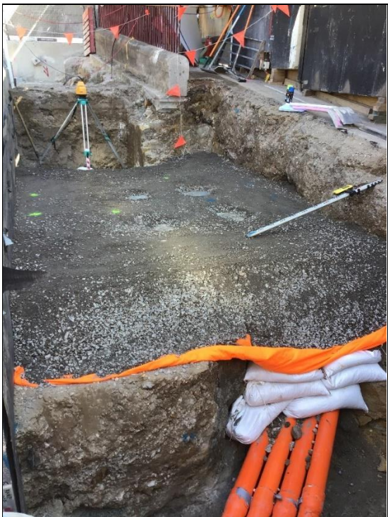
Figure 28 – Orange geofabric marker layer and imported roadbase from Boral Seaham quarry beneath electrical kiosk north of the Education Building (25 September 2020 – supplied by Built)
