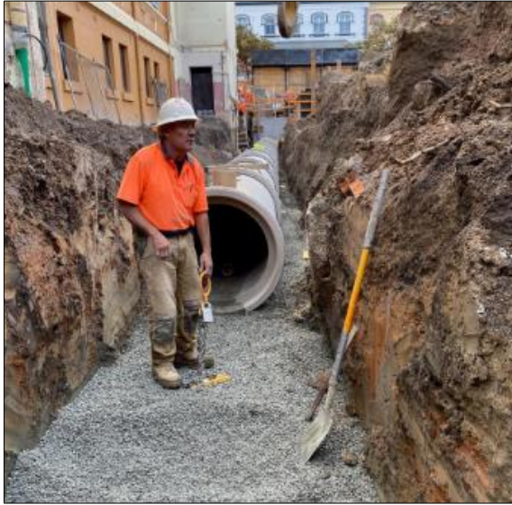
Figure 1: Pipe installation well within natural underling clays looking north (provided by Built Pty Ltd)
