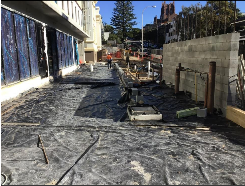
Figure 9 – Black plastic marker layer beneath concrete pavement on northern (front) side of Student Accommodation Building (26 June 2021 – supplied by Built)
