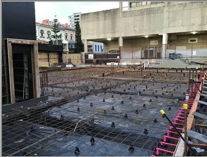
Figure 4 - Black plastic marker layer beneath Student Accommodation Building concrete slab (30 July 2020 - supplied by Built)
