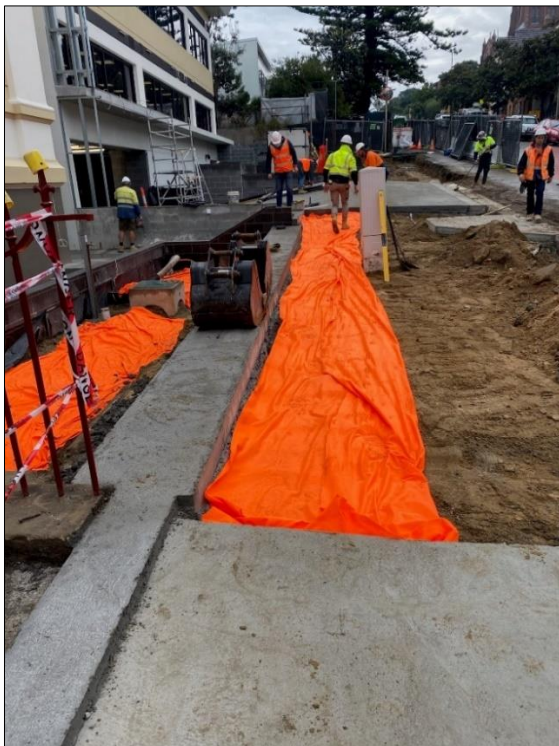
Figure 24 – Orange geofabric marker layer beneath the asphalt pavement along northern (front) boundary adjacent to footpath (19 July 2021 – supplied by Built)
