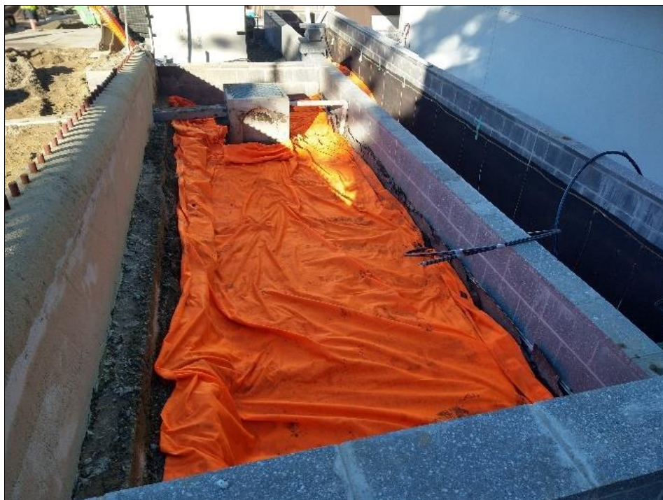
Figure 20 – Orange geofabric marker layer in garden beds at the front of the Education Building (16 July 2021)
