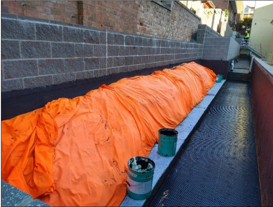
Figure 14 – Orange geofabric marker layer over impacted soils in garden bed and black geogrid matting beneath garden beds (over concrete) to rear of central building (13 July 2021)
