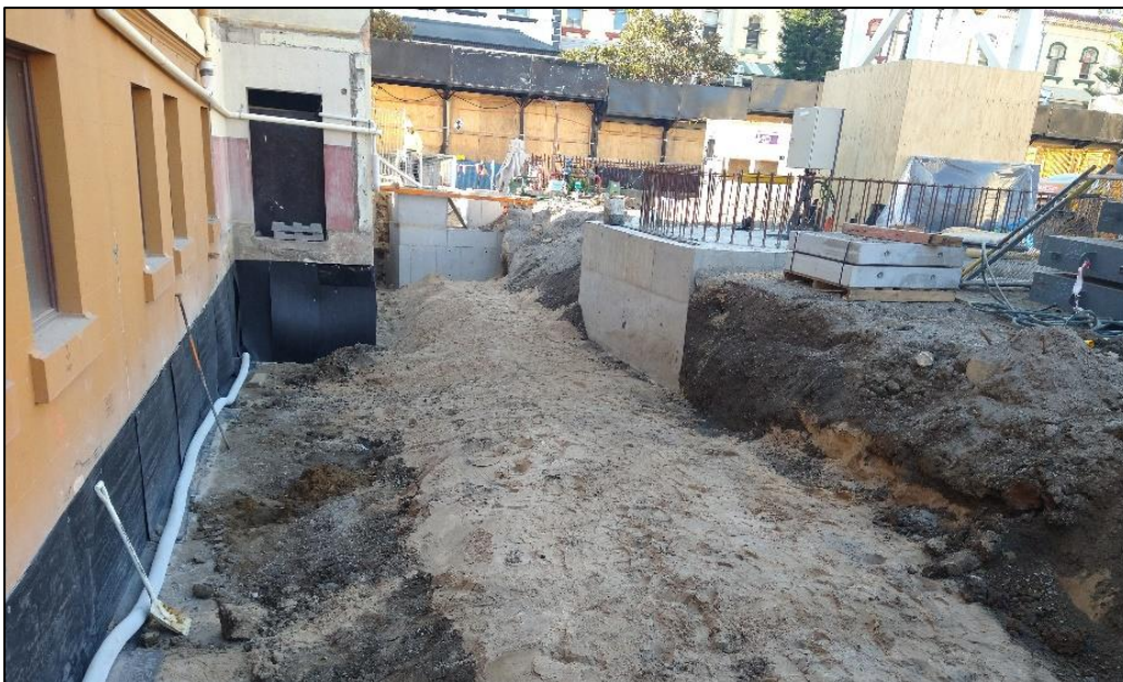
Figure 3: Imported “clean” sand over stormwater pipe looking north (building B on the left) (provided by DP – 3 July 2020), current trench condition.
