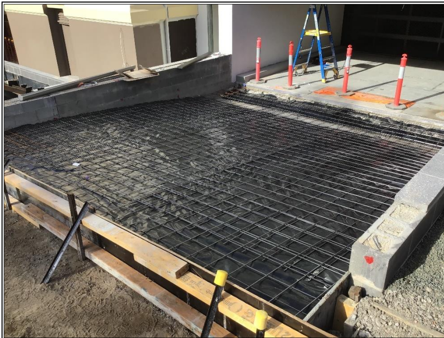
Figure 10 - Black plastic marker layer beneath driveway entrance concrete slab to Education Building carpark (6 July 2021 - supplied by Built)
