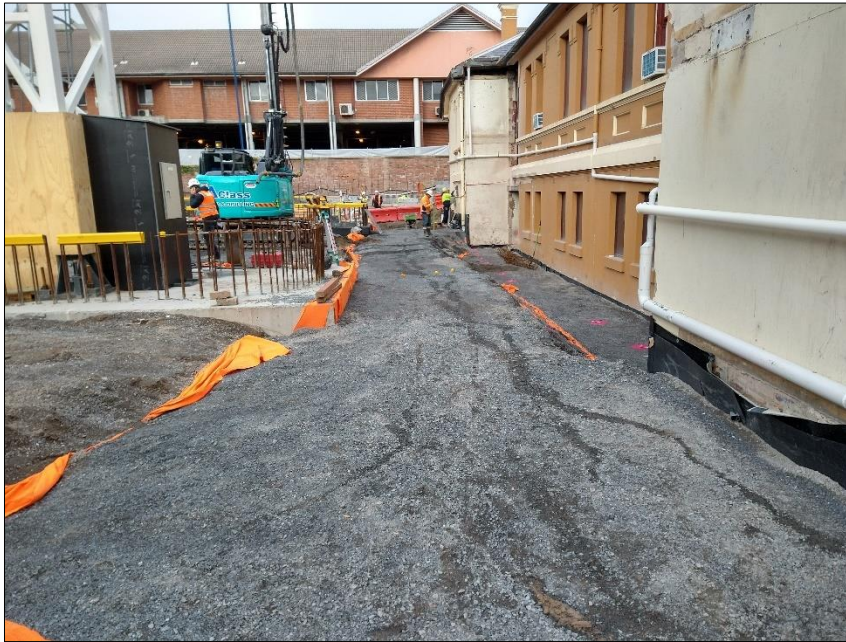
Figure 3: Imported fine crushed rock placed over orange geofabric marker layer placed over pipe backfill looking south (provided by Built Pty Ltd) (16 July 2020)
