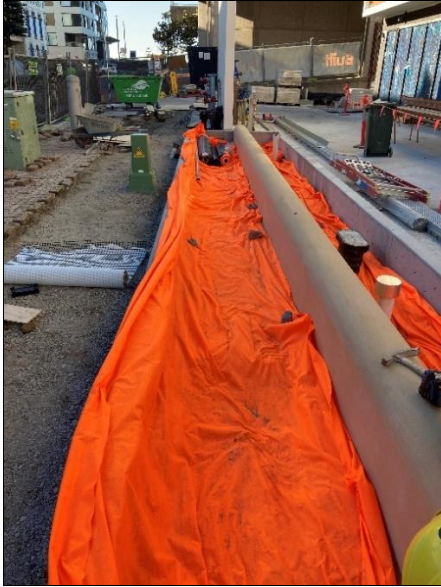
Figure 25 – Orange geofabric marker layer within garden bed on northern (front) side of the Student Accommodation Building (22 July 2021 – supplied by Built)
