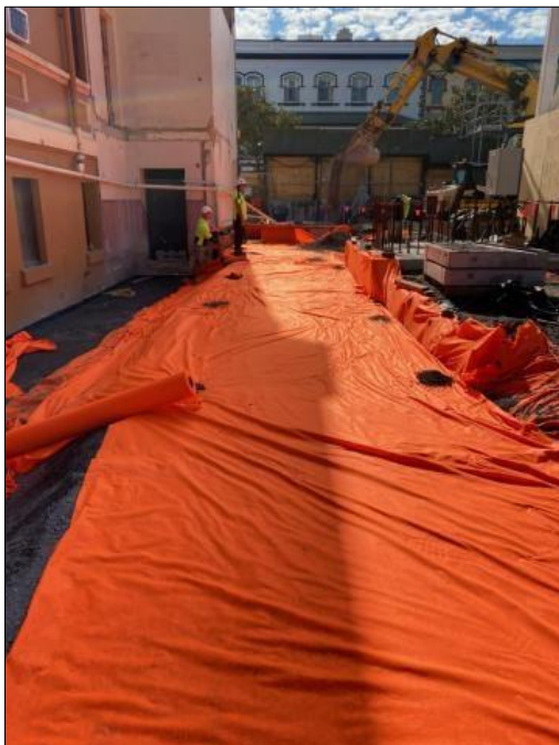
Figure 2: Orange geofabric sacrificial marker layer placed over pipe backfill looking north (provided by Built Pty Ltd) (16 July 2020)
