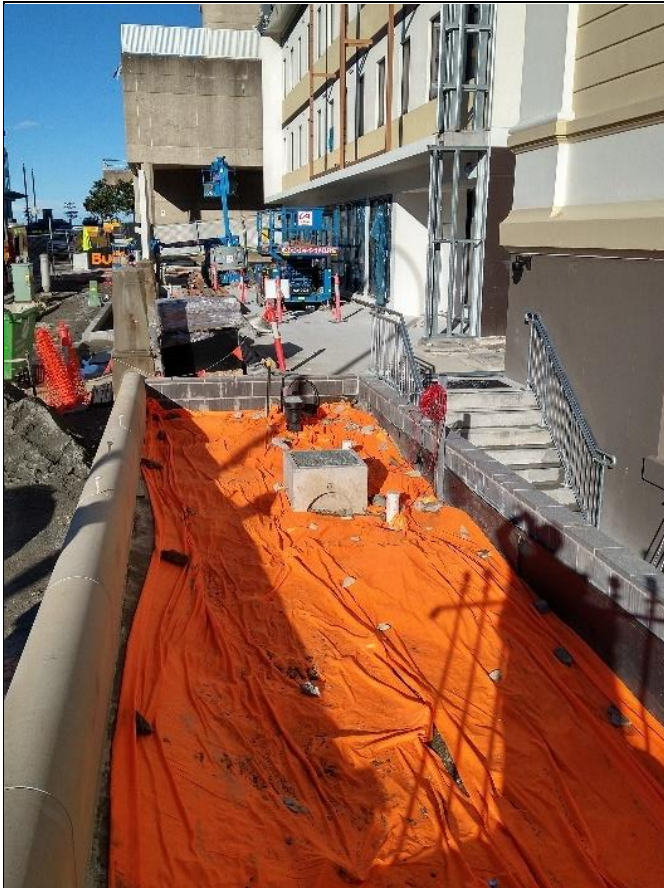
Figure 21 – Orange geofabric marker layer in garden beds at the front of the central building (16 July 2021)
