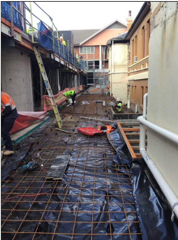
Figure 5 - Black plastic marker layer beneath Atrium concrete slab (25 August 2020 - supplied by Built)
