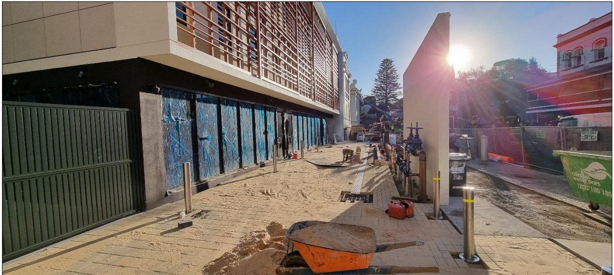
Figure 33 – Sand from Saddingtons (Mackas Sand & Soil - Williamtown quarry) used as paving sand at front of Student Accommodation building (28 July 2021 – supplied by Built). Pavers laid over packing sand (from Saddingtons) over concrete.
