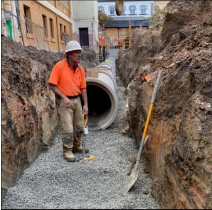
Figure 2: Pipe installation well within natural clays looking north (provided by Built Pty Ltd)
