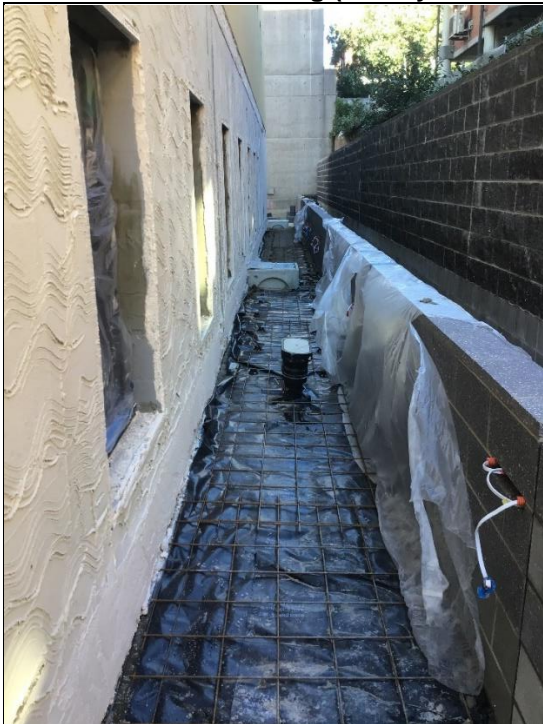
Figure 13 – Black plastic marker layer beneath concrete/crushed granite paths to rear of Student Accommodation Building (17 May 2021 - supplied by Built)
