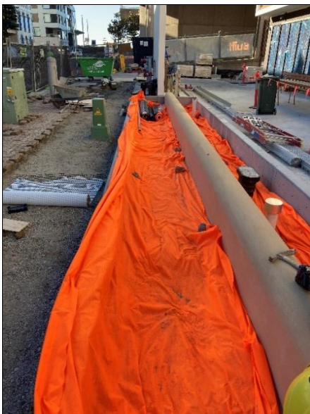
Figure 24 – Orange geofabric marker layer within garden bed on northern (front) side of the Student Accommodation Building (22 July 2021 – supplied by Built)
