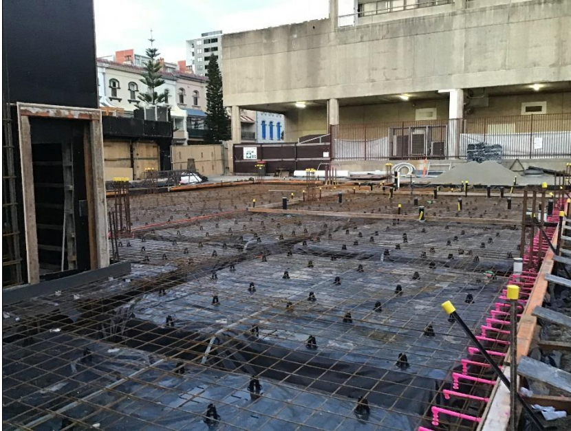
Figure 25 - Black plastic marker layer beneath Student Accommodation Building concrete slab (30 July 2020 - supplied by Built)
