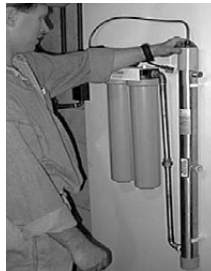
Install UV unit
