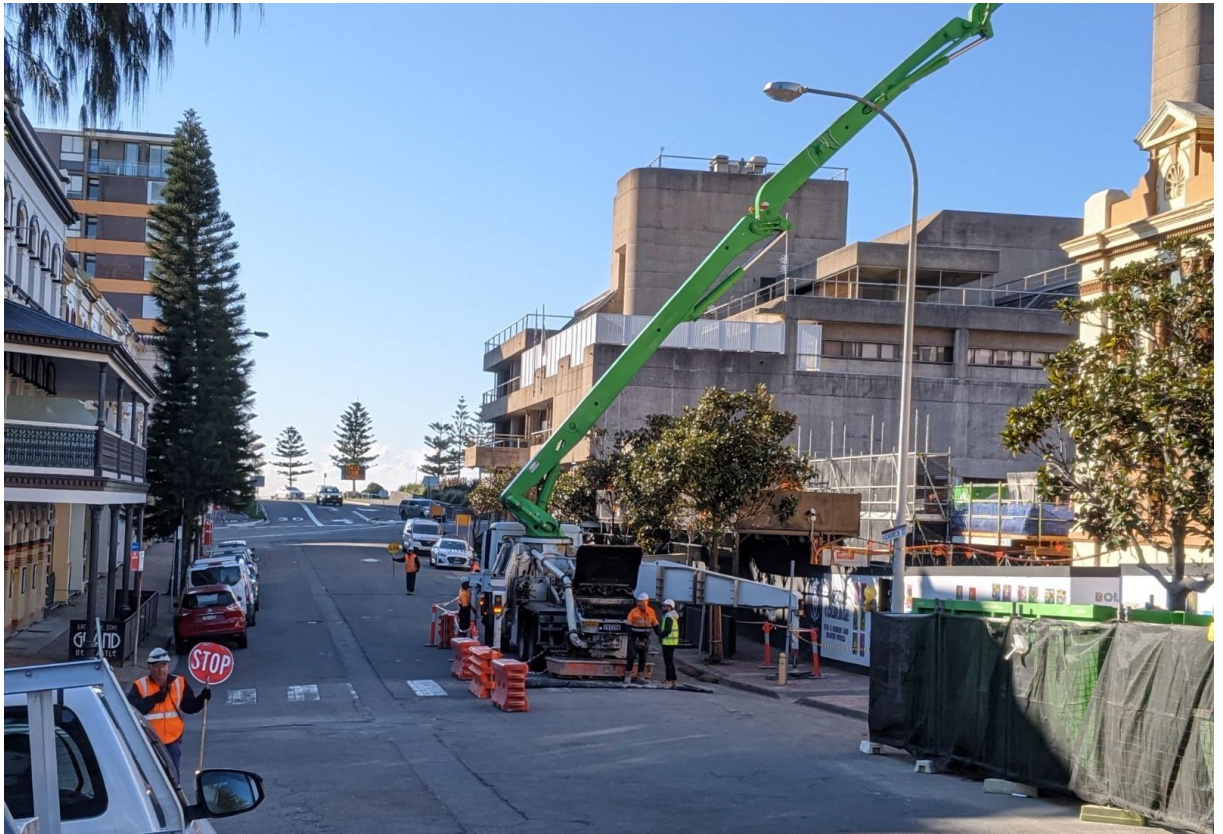
Crane operating on Church Street, with evidence of traffic control being implemented.
