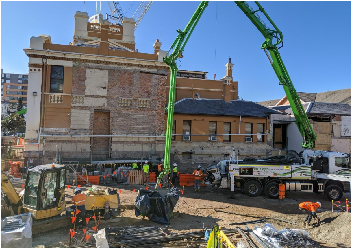
General construction area of the education building, with no dust generation observed as a result of works or stockpiling.
