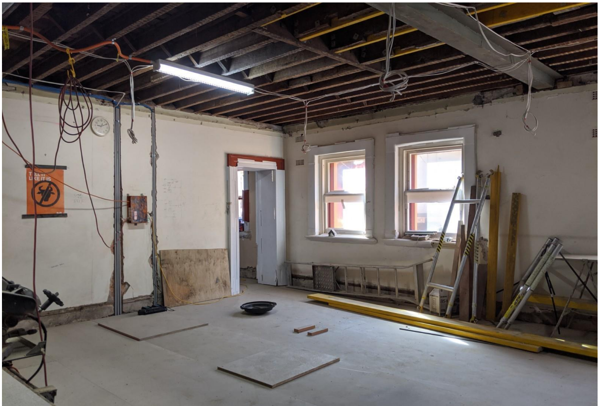
Construction works underway within the Courthouse building.
