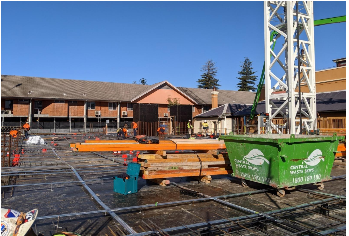
Construction works underway on the Residential building, with waste receptacles observed.
