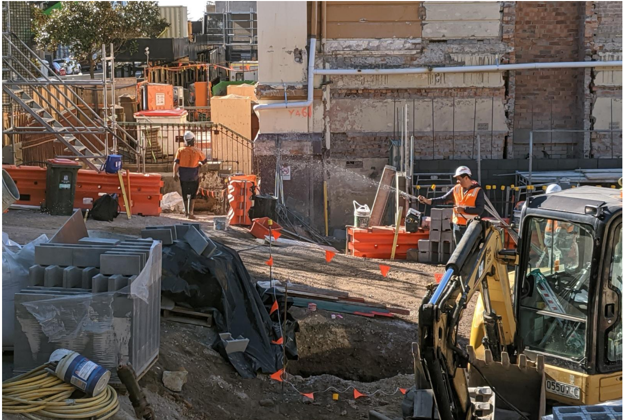
A construction worker spraying the access road to limit the potential for dust generation.
