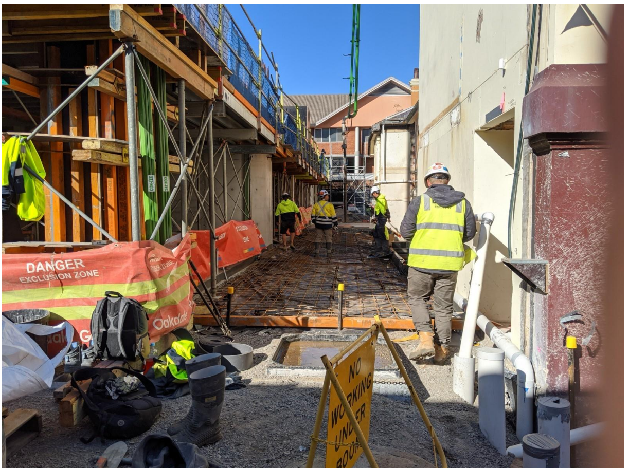
Concreting works between the Courthouse building and Residential Building (currently under construction).
