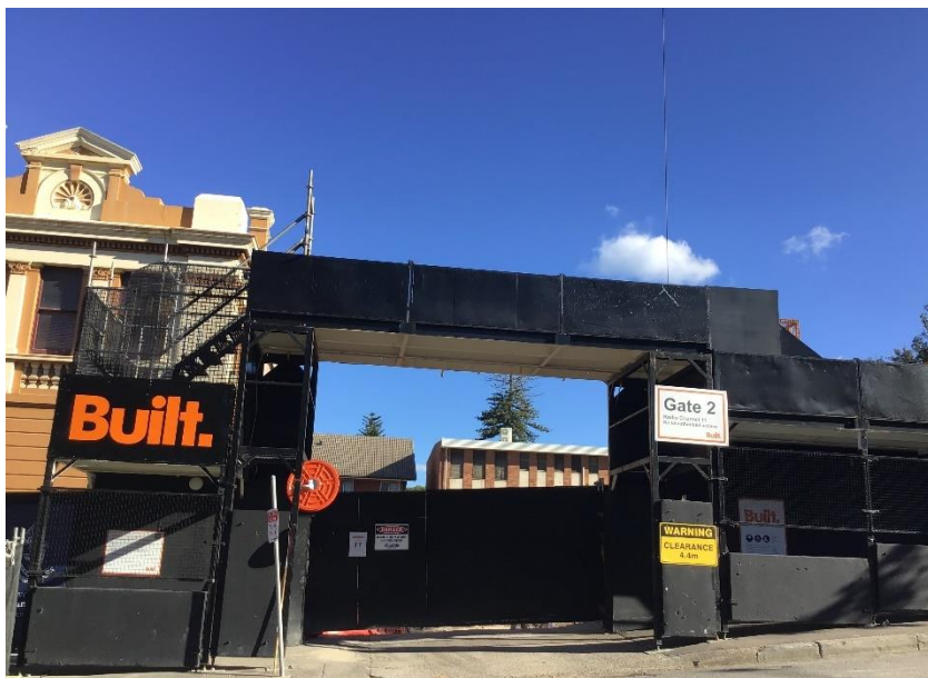
Figure 11: Building A – Gate 2 on Western end of Church Street
