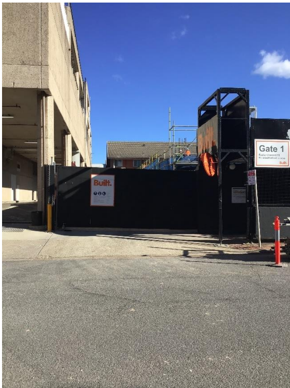
Figure 10: Building C - Gate 1 on Eastern end of Church Street
