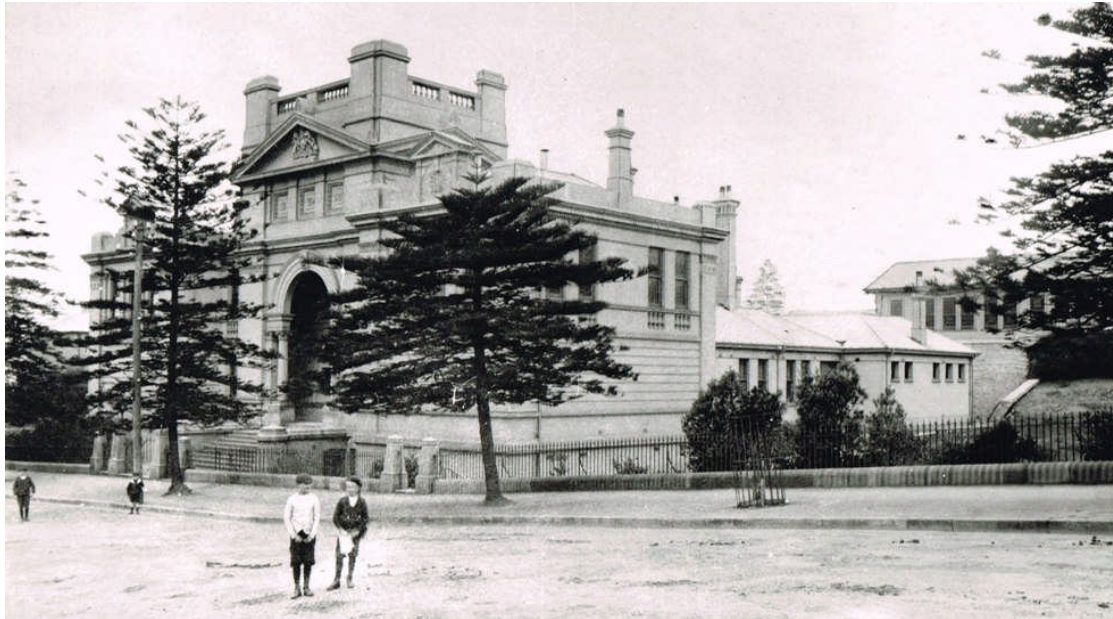
Plate 29: An early twentieth century photo of the 1892 Newcastle Court House. (Govt Printing Office No 1114)
