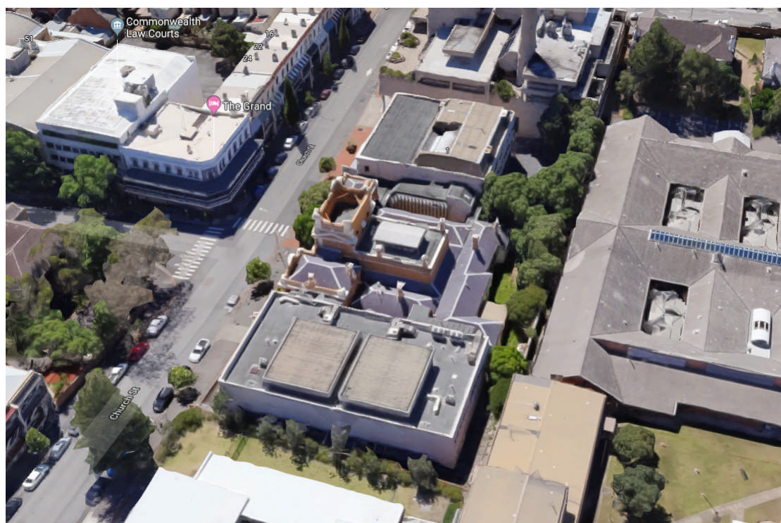
Plate 32: Aerial view of the Newcastle Courthouse complex from the west. (Google Maps)
