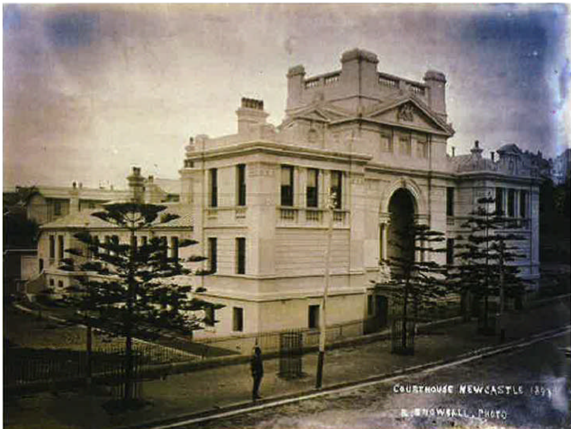
Plate 30: An 1893 photo of the 1892 Newcastle Court House by Ralph Snowball. (Hunter Photo Bank, ASGN0102-B4.)
