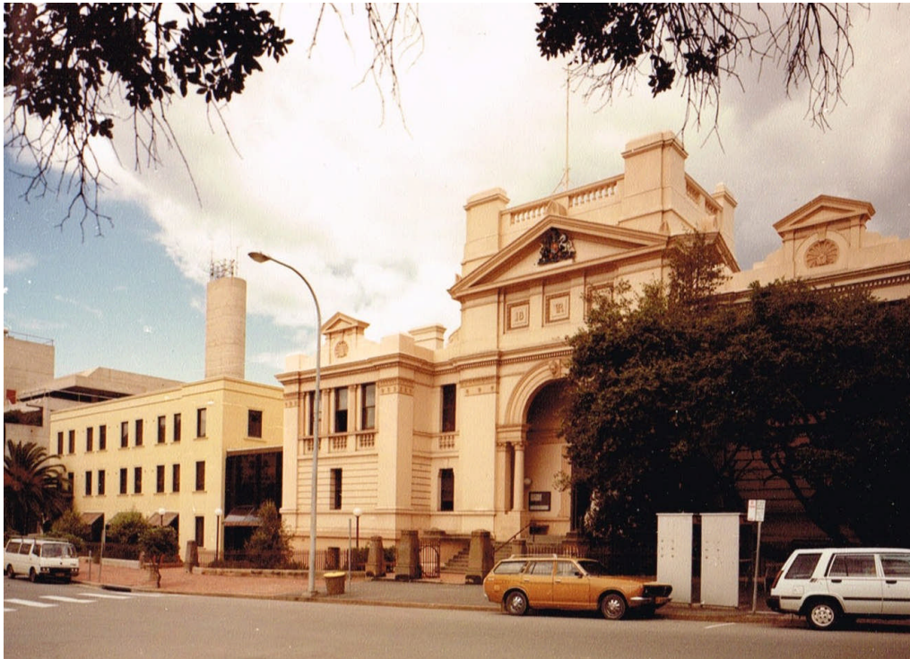
Plate 12: The Refurbished Administration block circa 1983. (John Lugg Public Works Photographer)
