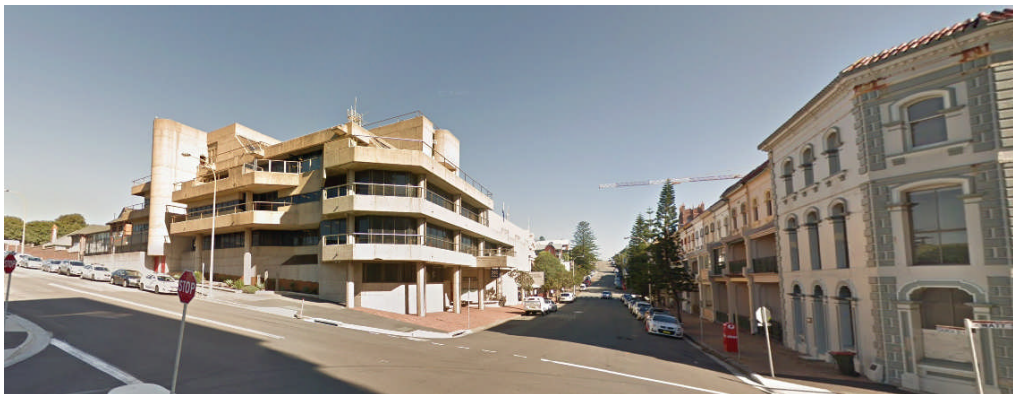
Plate 33: The 1984 Newcastle Police Station from the east. (Google Maps)
