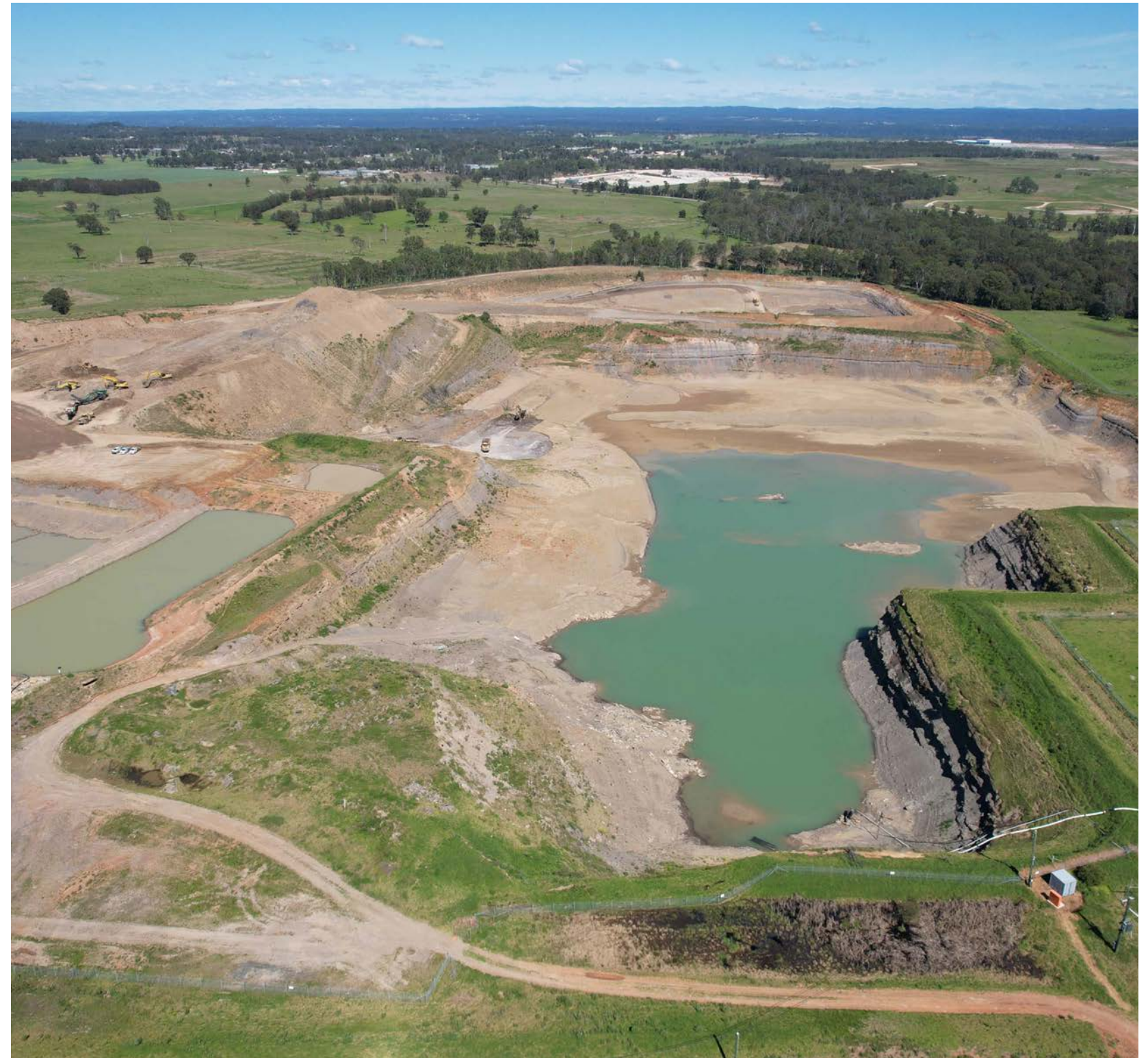
Figure 2 Aerial view of the existing site
