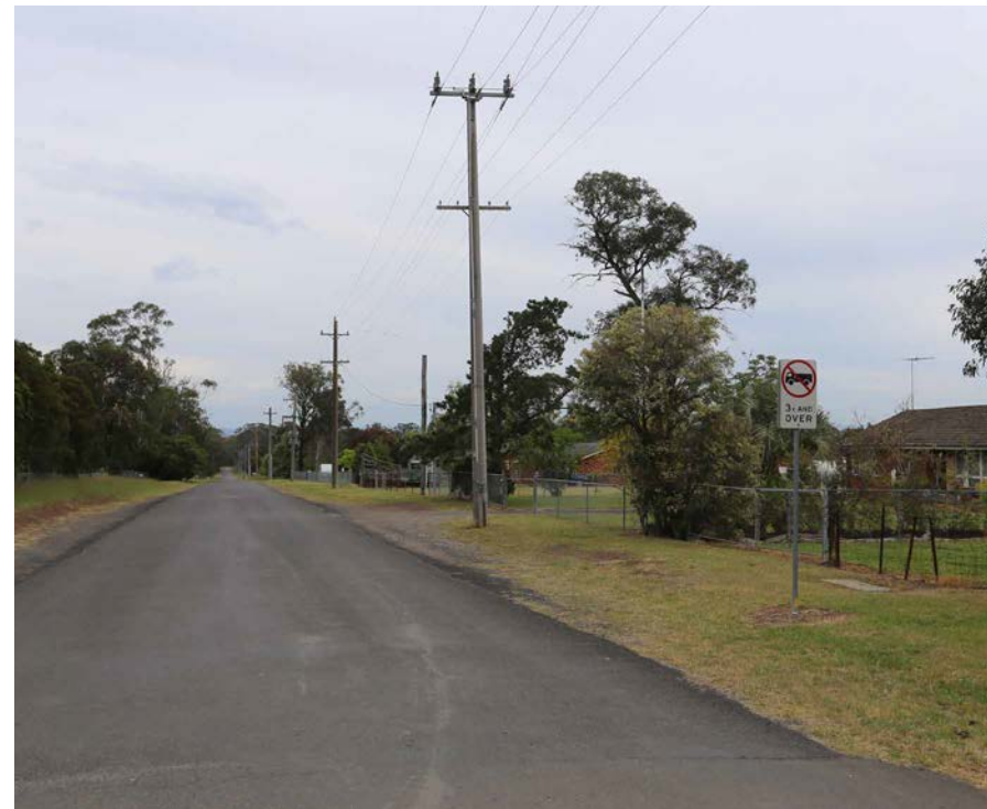
Photo 14. View west from intersection of Victor Ave and Western Road
