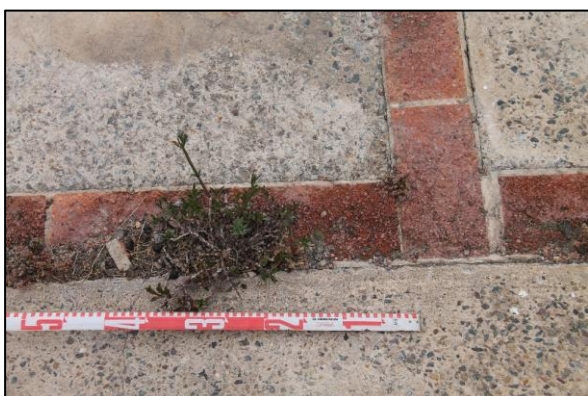
Figure 54. Detail of the brick feature in the location of former building no. 1
