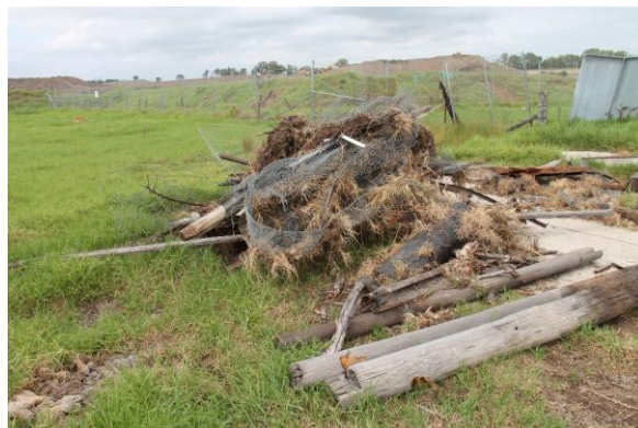
Figure 69. View of concrete features and demolished fencing in the location of former building no. 4, facing southeast
