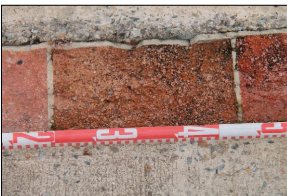
Figure 55. Detail of the brick feature in the location of former building no. 1
