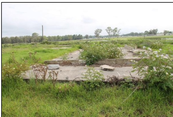
Figure 56. View of a concrete pad and low wall in the location of former building no. 1, facing north
