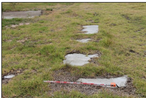
Figure 68. View of concrete features in the location of former building no. 4, facing south
