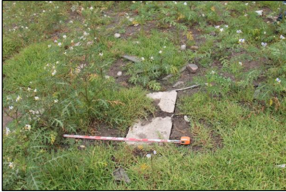
Figure 62. View of a concrete feature in the location of former building no. 2, facing west
