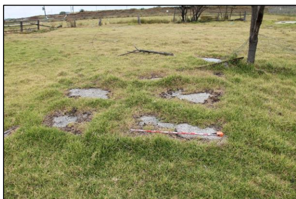
Figure 89. View of a concrete surface in the location of former building no. 6, facing north
