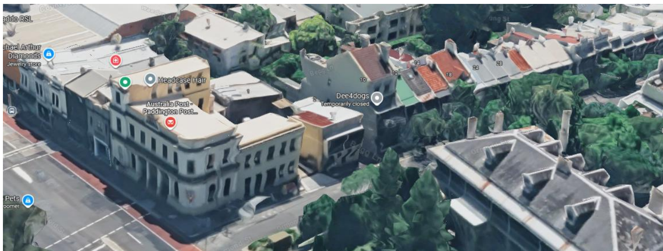
Figure 5 Oblique aerial of the Paddington Post Office 88 Oxford Street (corner of Oxford Street and Ormond Street) which is a tall building on a street corner adjacent to two storey terraces
