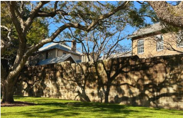
Figure 11 Victoria Barracks Perimeter Wall
